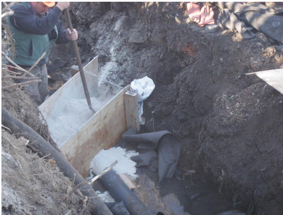
Installation of discharge piping through 2' bentonite dam
