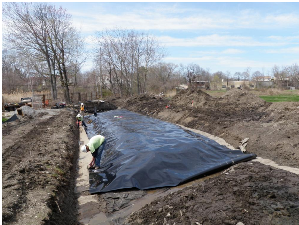
Landfill cap repair above leachate discharge piping
