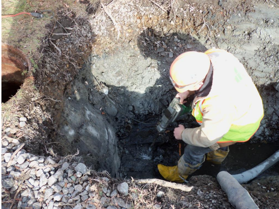
Concrete footing discovered at base of WCDEF sanitary manhole
