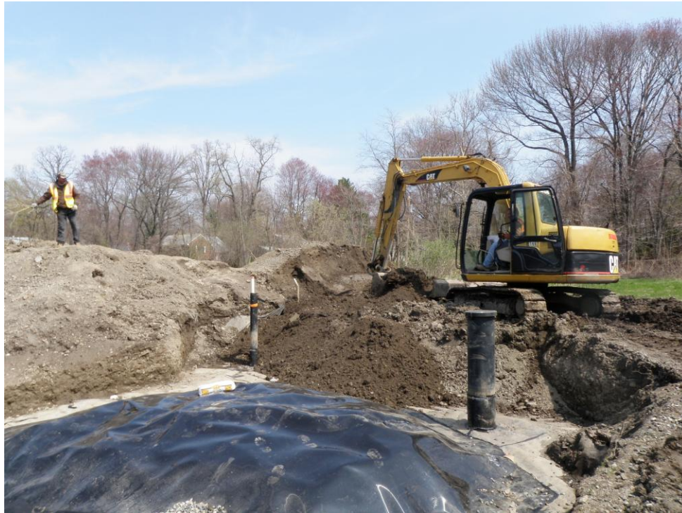
Backfilling discharge trench in vicinity of leachate recovery well
