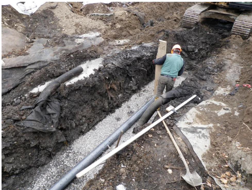
Installation of perforated 6" discharge piping
