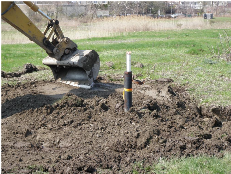
Backfilling and grading around Piezometer
