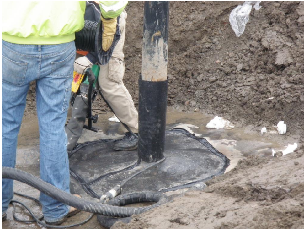
Boot construction around Piezometer (typ)
