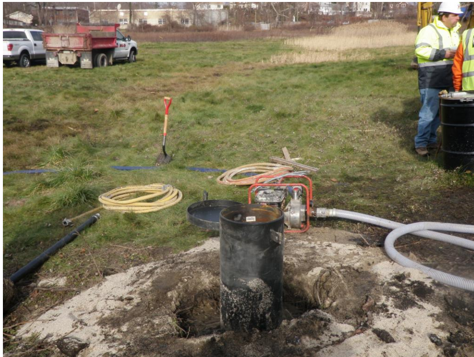
Leachate Recovery Well Installation
