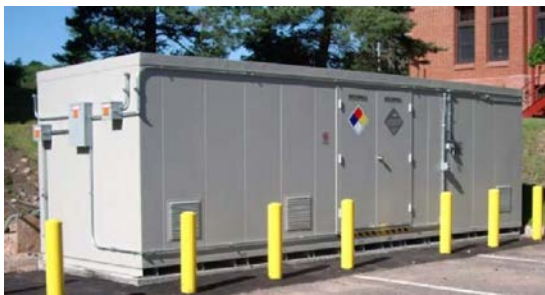
FIGURE 7-1. Typical Hazardous Waste Storage Building
