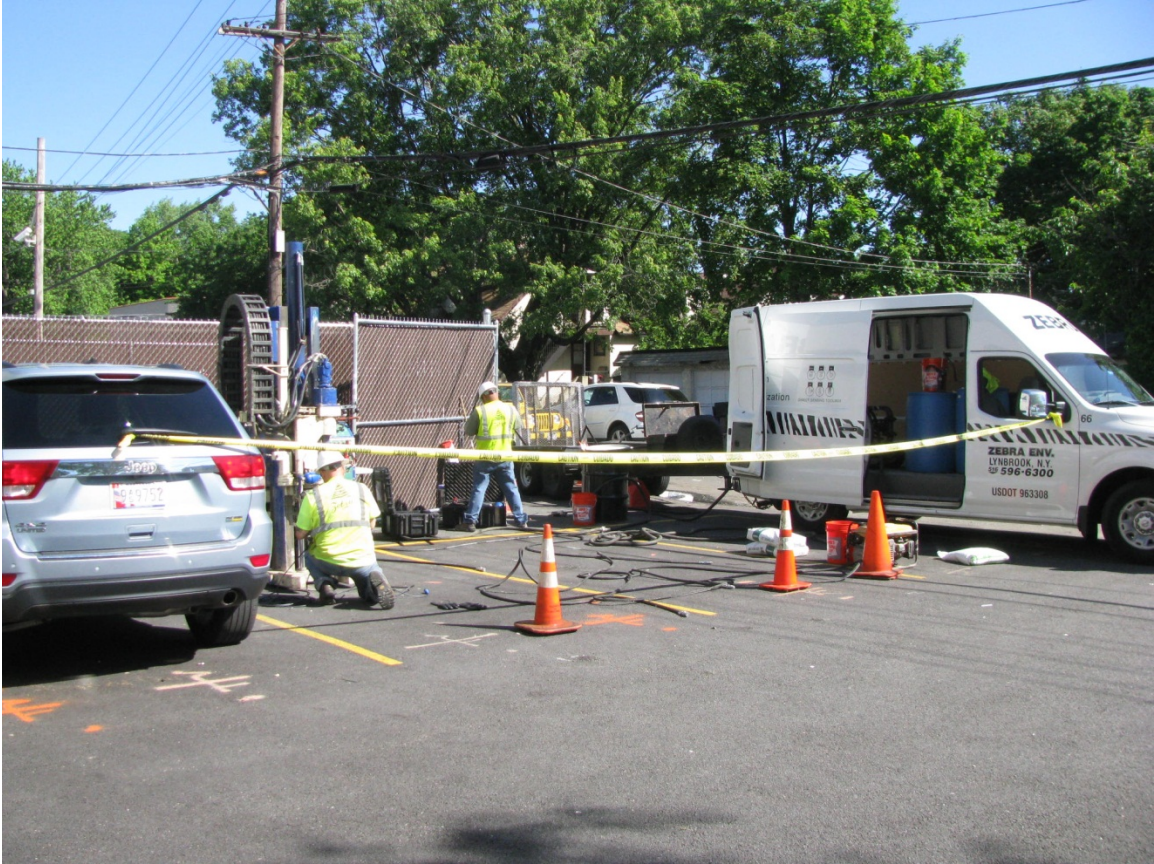
PHOTOGRAPH OF REMEDIAL INJECTIONS COMPLETED IN 2014 IN THE VICINITY OF MONITORING WELL MW-02.
