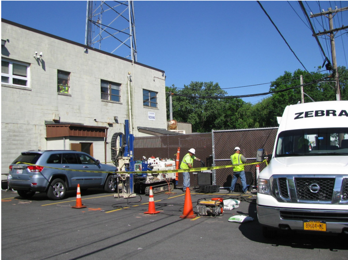
PHOTOGRAPH OF REMEDIAL INJECTIONS COMPLETED IN 2014.
