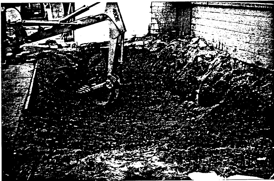
Backhoe leveling off excavation pit.
