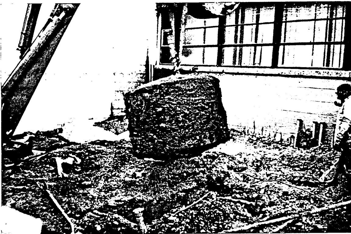
The removal of Tank #3 (275-gallon UST) from the excavation pit.
