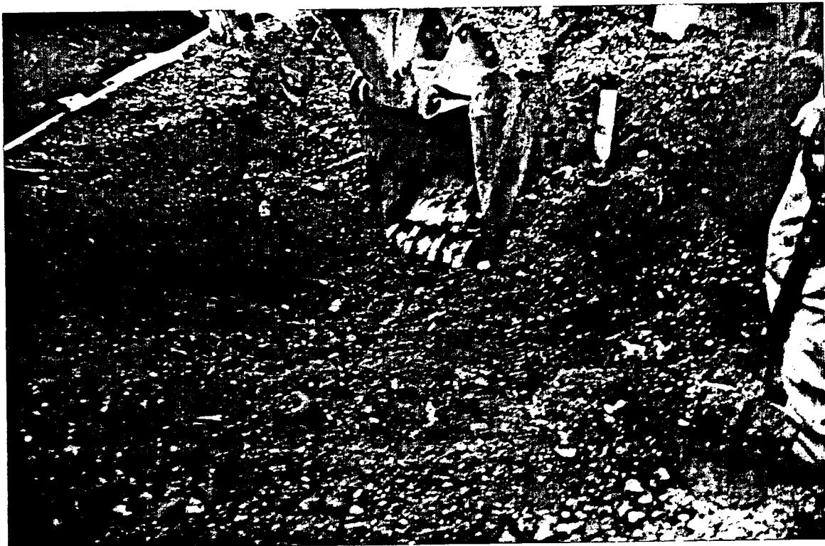
Backhoe excavating the UST area to determine actual number of tanks.
