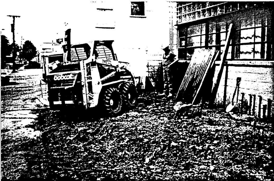
Bobcat clearing UST area of all rocks before excavation activities begin.
