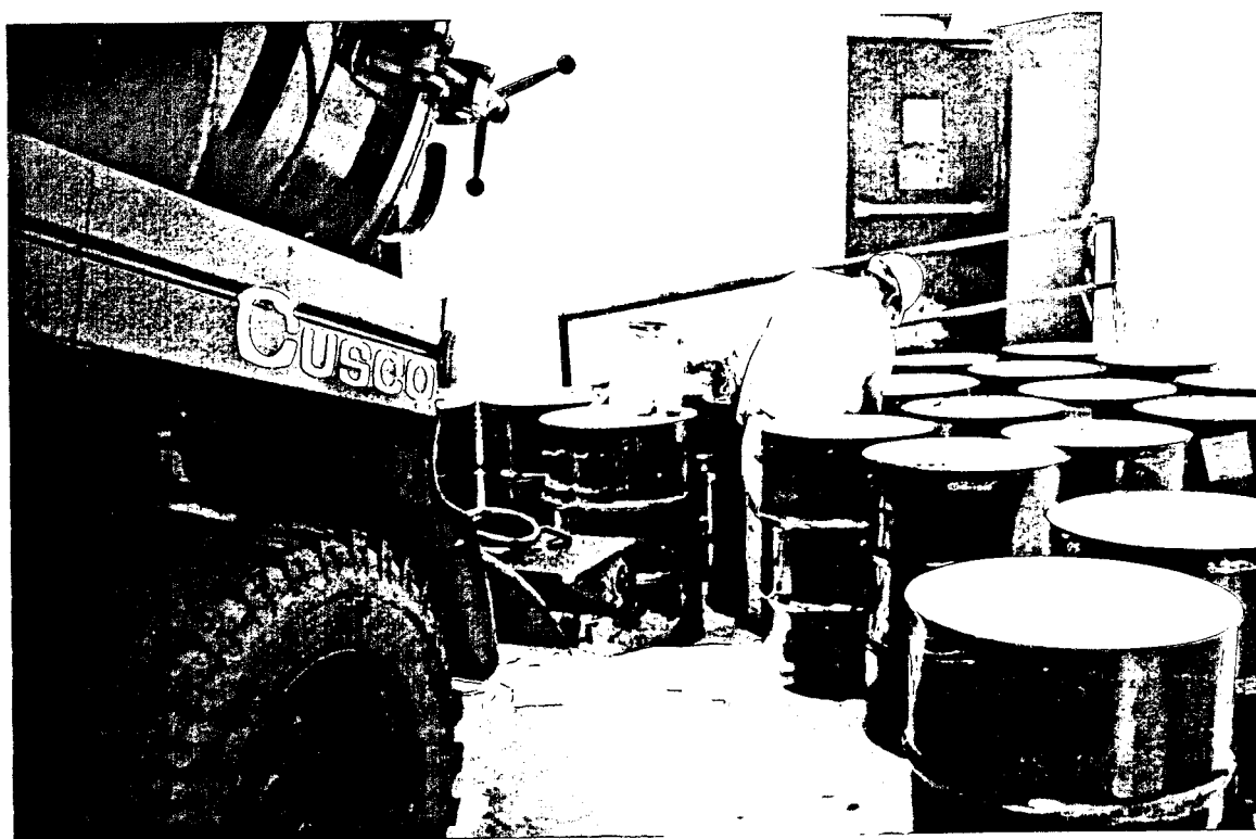
Vacuum truck, provided by Environmental Products and Services, Inc., transfers UST contents into 55-gallon drums.
