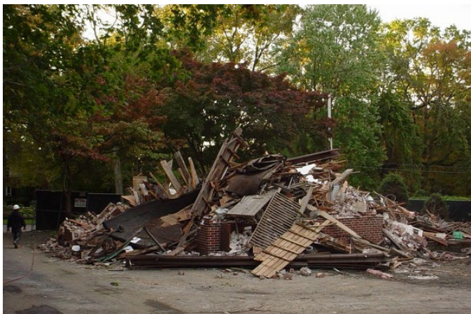
55 Hillandale Post Demolition (source: https://response.epa.gov/site/site_profile.aspx?site_id=1600 )
