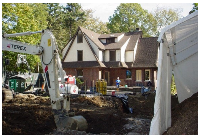
55 Hillandale before demolition (source: https://response.epa.gov/site/site_profile.aspx?site_id=1600 )
