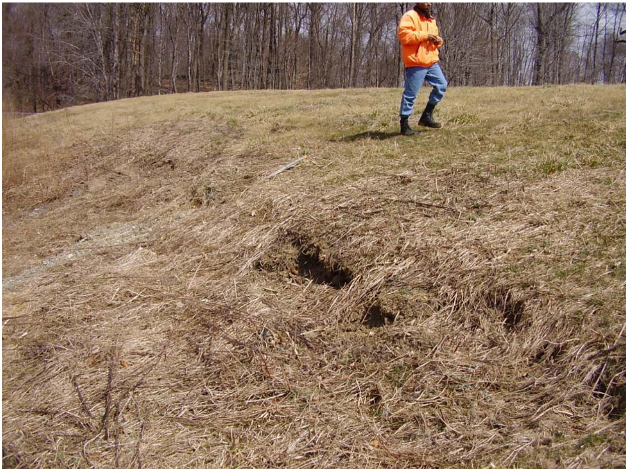
Place seeded topsoil on the eroded area on the western side of the landfill
