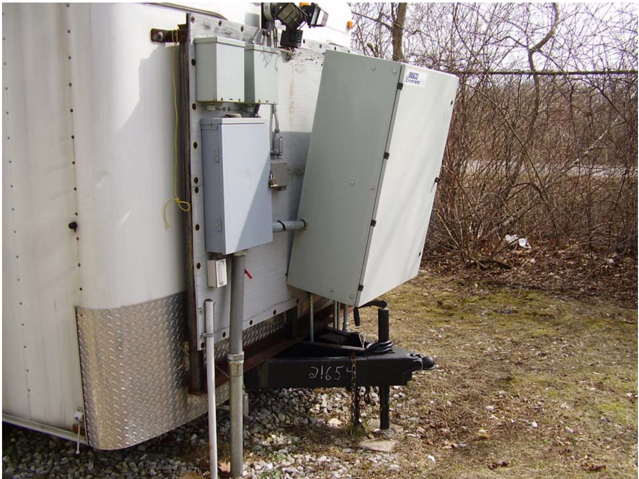
Reattach electrical panel on the remediation trailer
