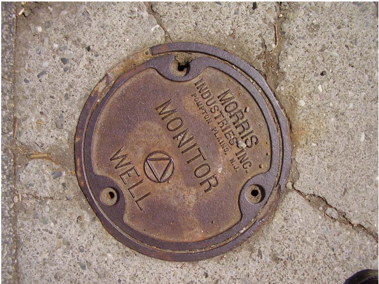
Replace missing bolts from well caps
