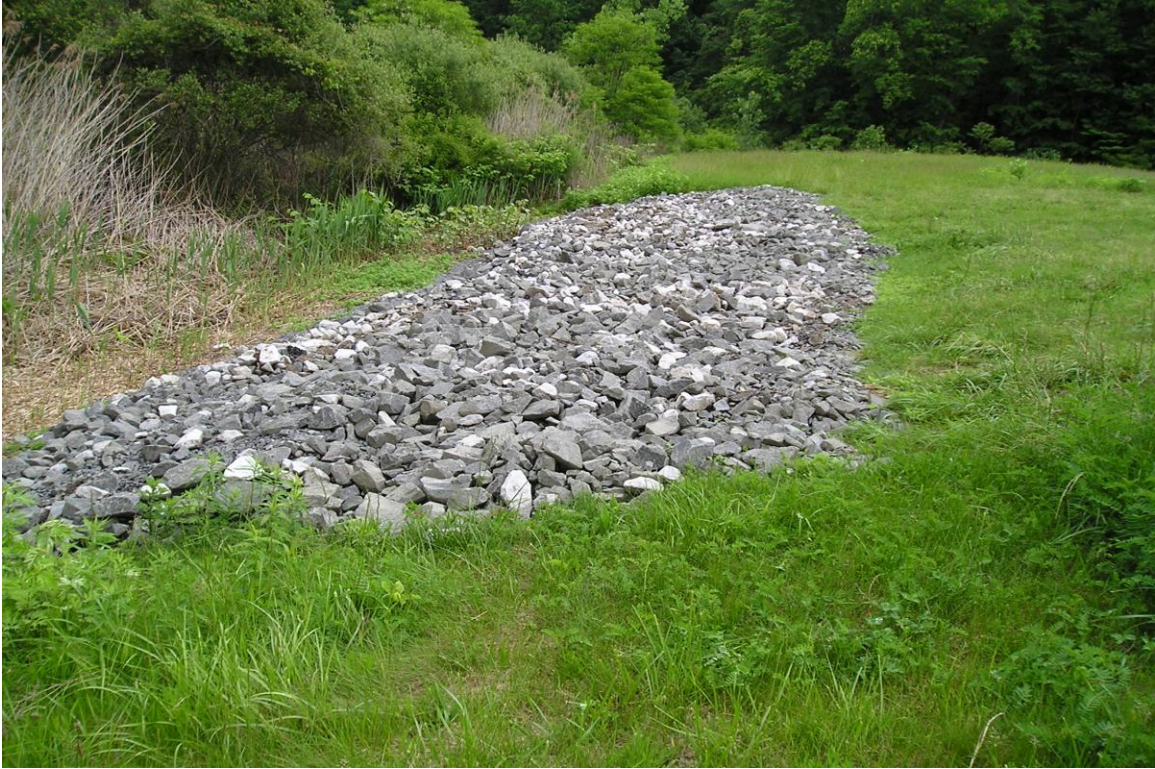
Photo 23: West slope erosion area repair (looking north)
