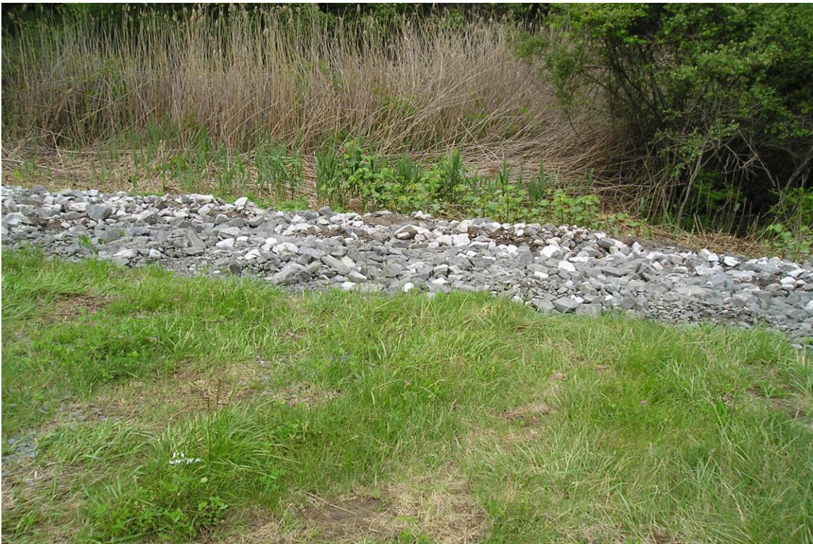
Photo 22: West slope erosion area repair (looking west)
