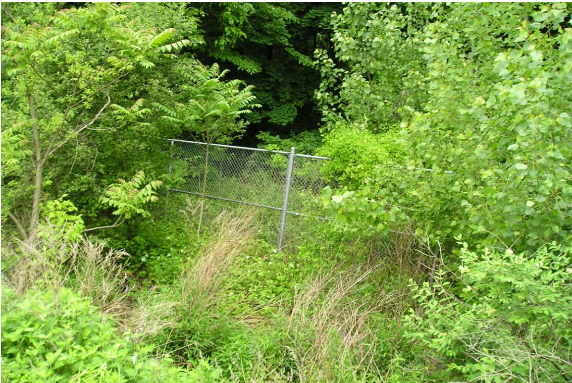
Photo 18: Fallen tree repair on north fence (mid section)
