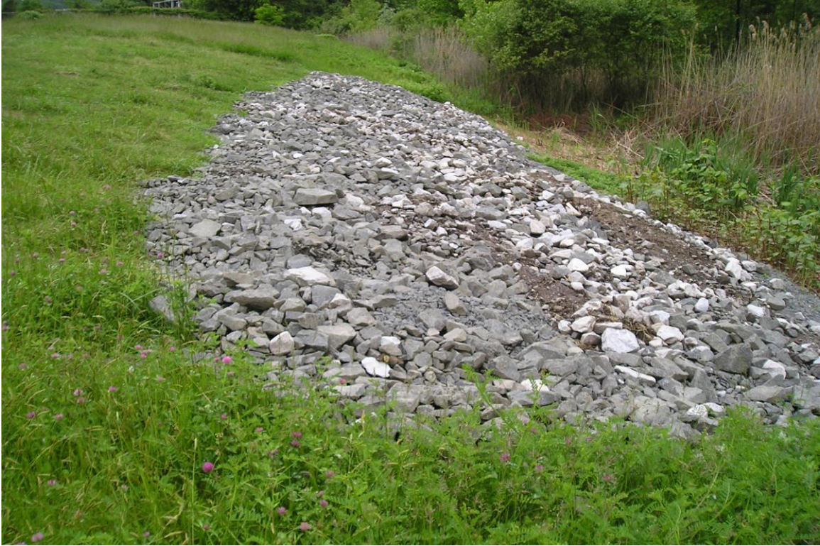
Photo 21: West slope erosion area repair (looking south)
