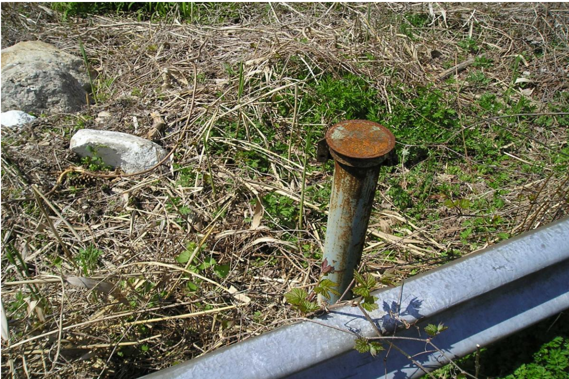
Photo 10: Well MW-12 (lock missing)
