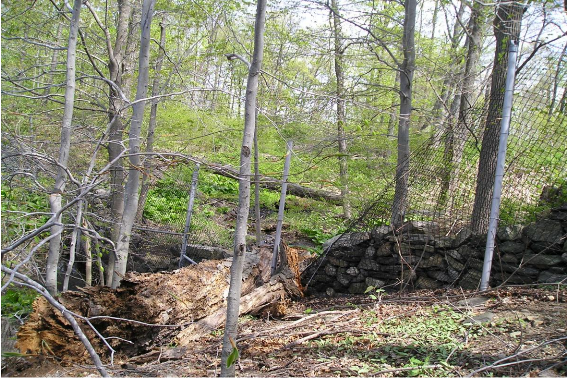
Photo 17: Another view of fence damage by large, rotten tree near stream inlet
