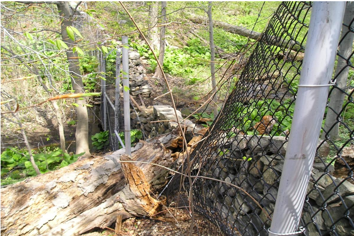
Photo 16: Fence damage by fallen tree (near stream inlet – northeast of landfill cap)
