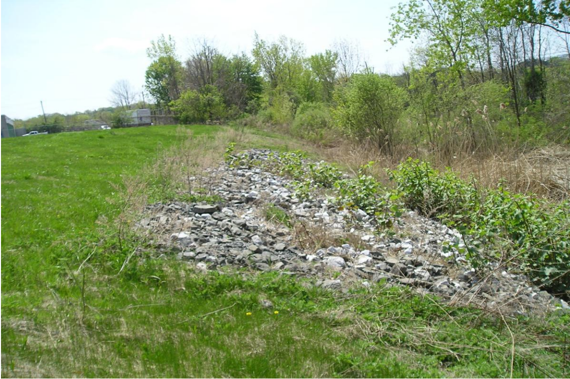
Photo 19: West slope erosion area repair (looking south)
