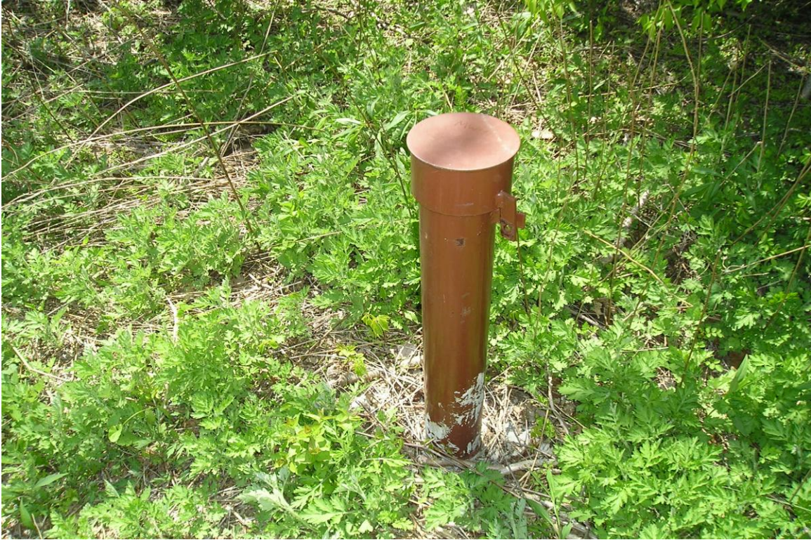
Photo 9: Well MW-11 (lock missing)
