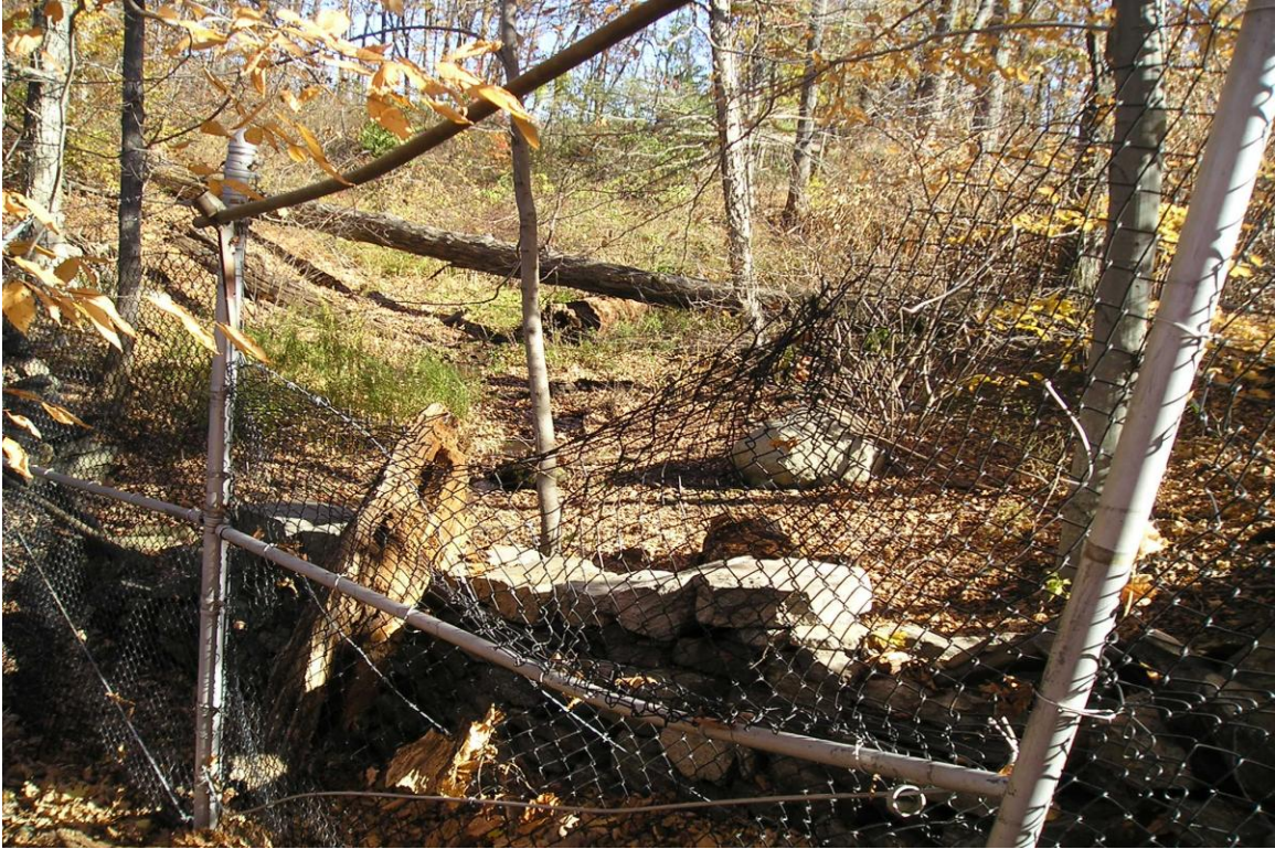
Photo 17: Fence partially repaired (near stream inlet)
