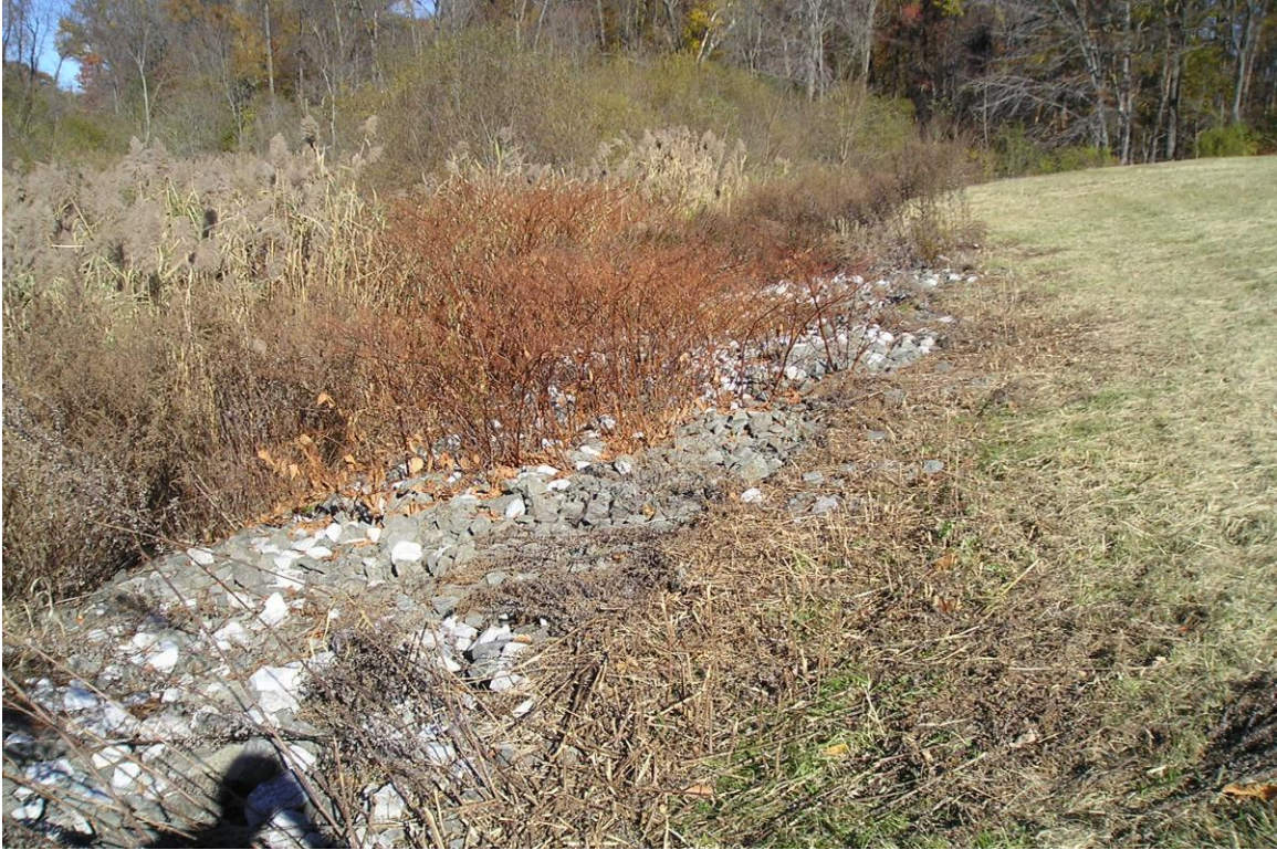
Photo 19: West slope erosion area repair (looking north)
