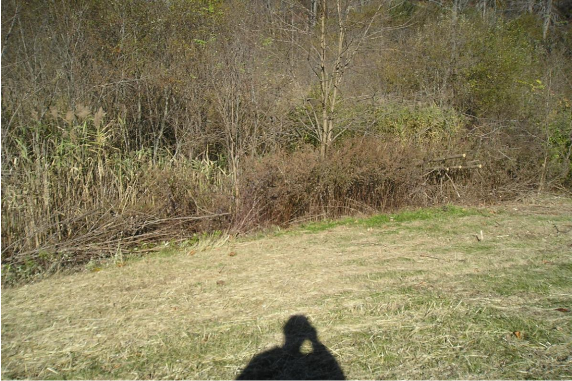
Photo 23: Downed tree removed from northwestern portion of landfill cap.
