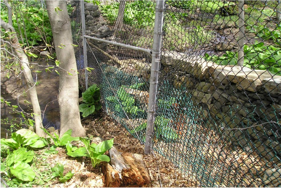
Photo 17: Fence repaired (near stream inlet)
