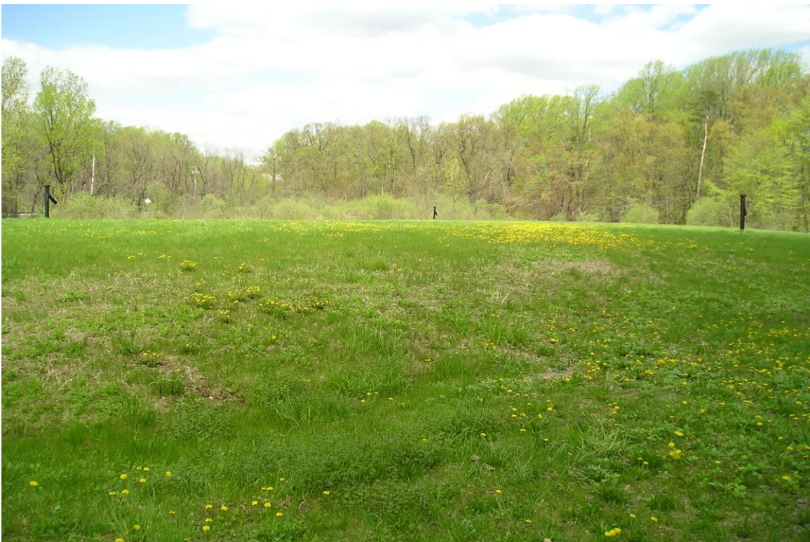
Photo 14: Grass on landfill cap
