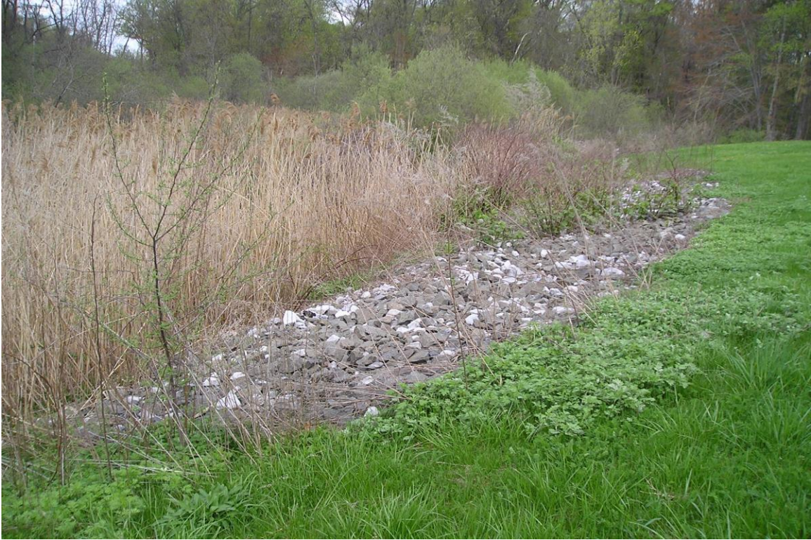
Photo 19: West slope erosion area repair (looking north)
