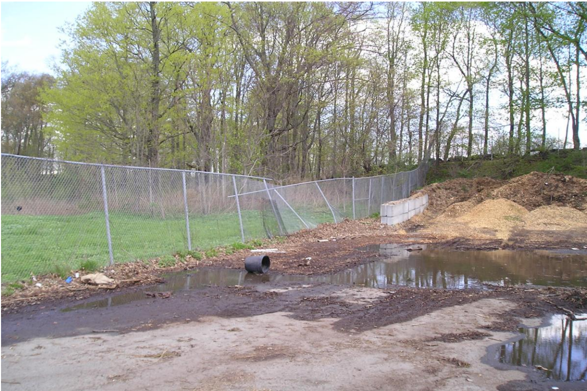
Photo 18: South fence damage (looking east)
