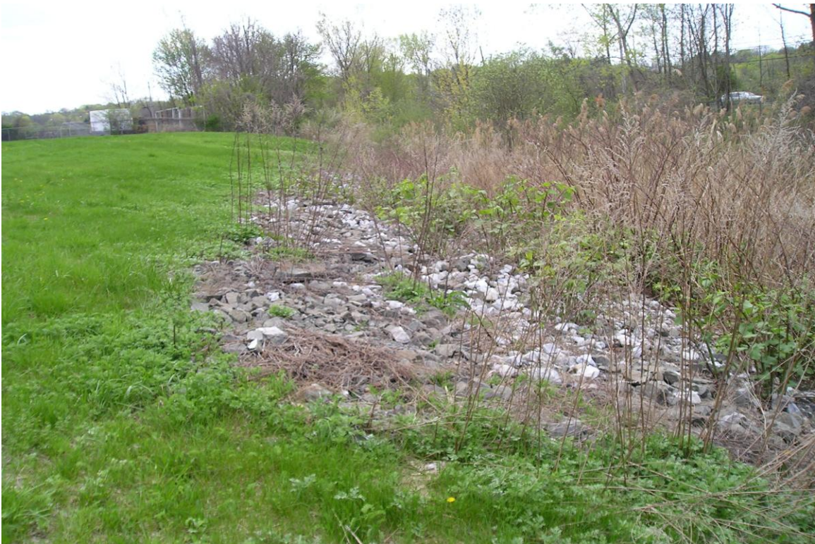
Photo 20: West slope erosion area repair (looking south)
