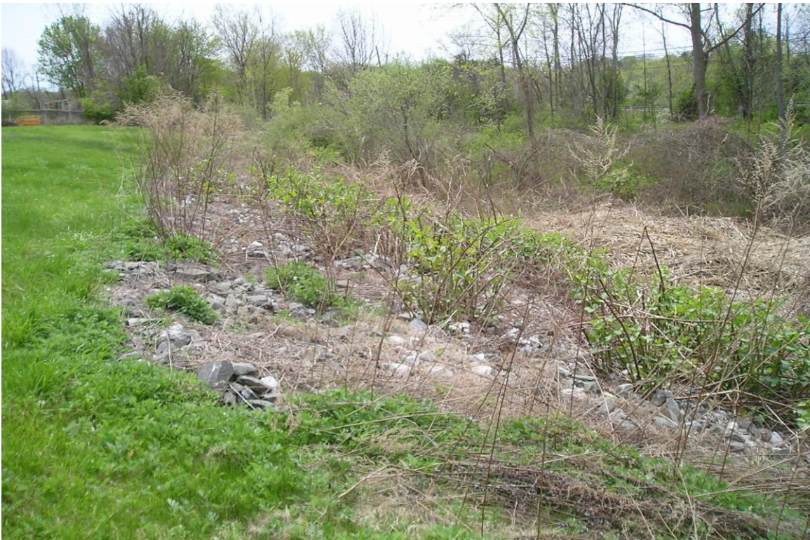
Photo 14: West slope erosion area repair (looking south)
