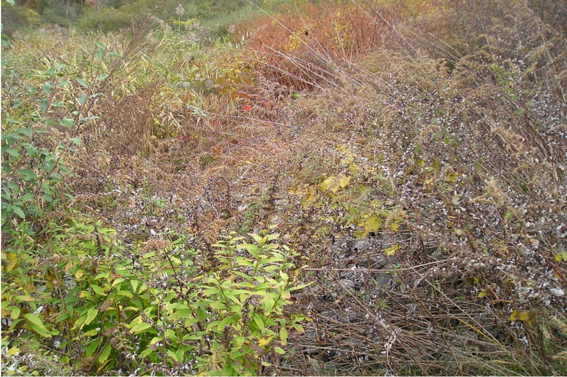
Photo 13: West slope erosion area repair (looking north)
