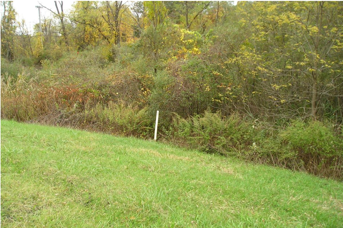
Photo 10: Grass on landfill cap
