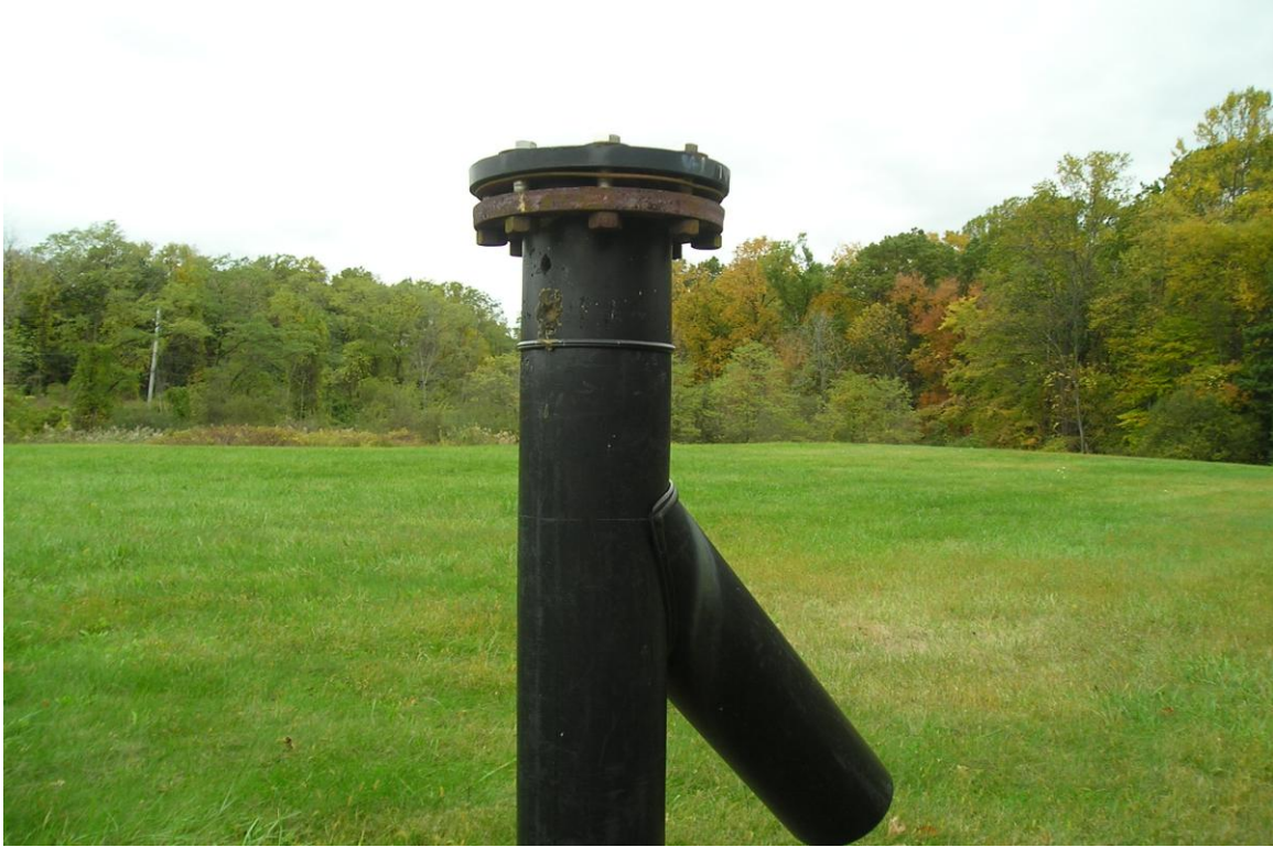
Photo 1: Vent V-1 (eraser size hole).
