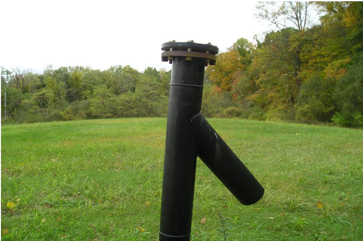
Photo 2: Vent V-2 (quarter size hole near top).
