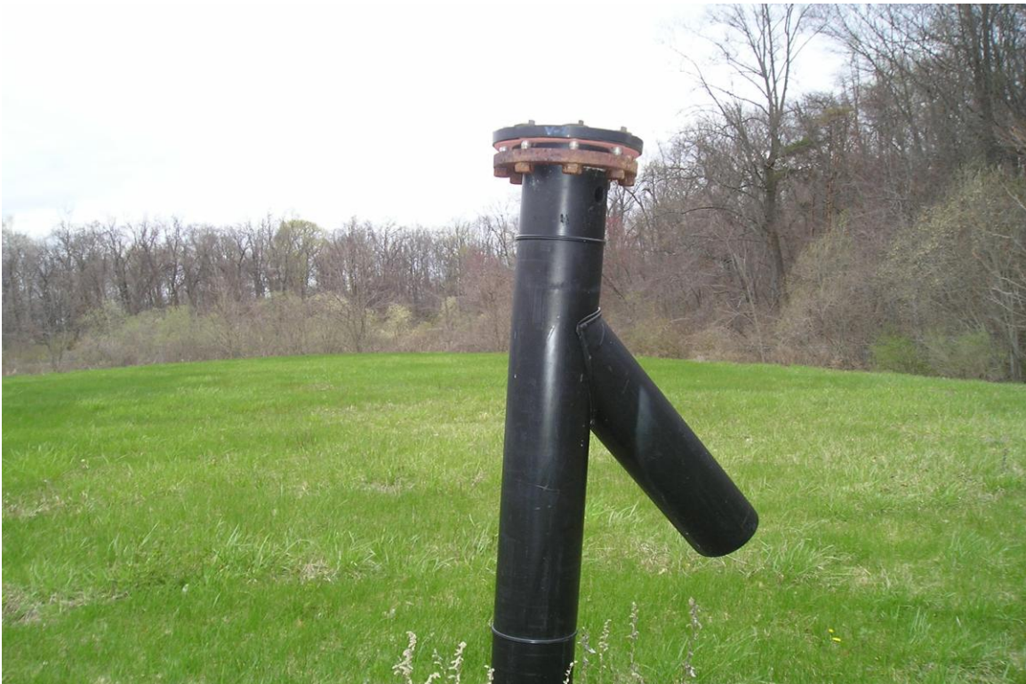
Photo 2: Vent V-2 (quarter-sized hole near top)
