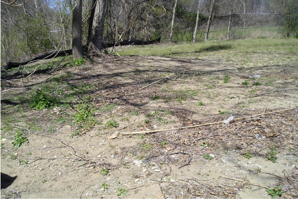
Photo 17: Bare areas and collapsed silt fence in front of the facility
