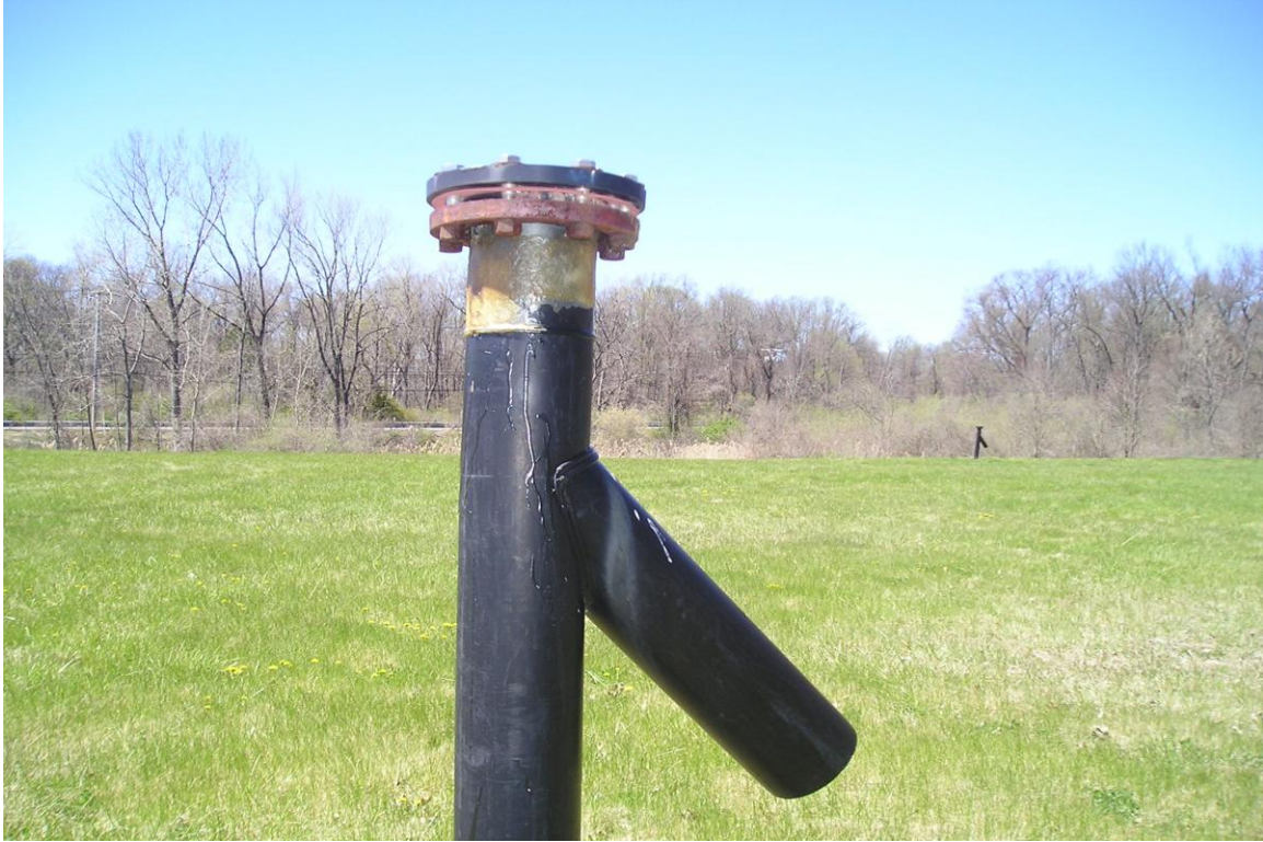
Photo 1: Vent V-1 (hole repair shown)
