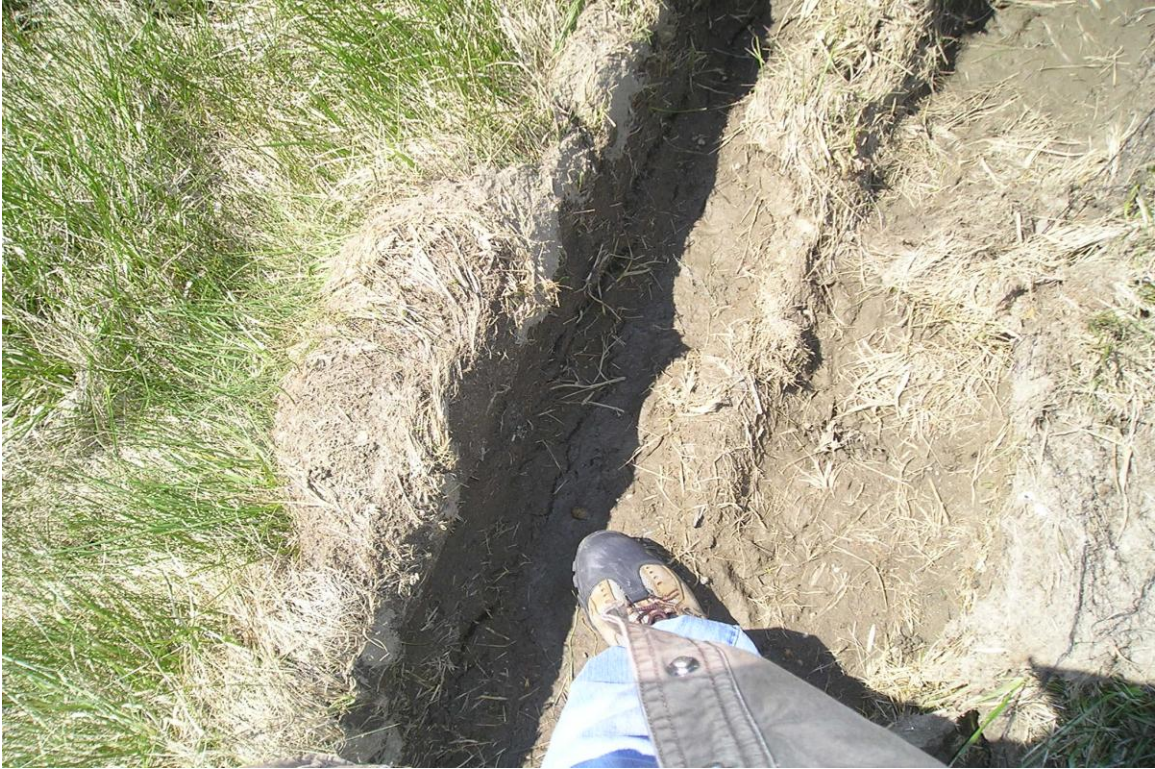
Photo 15: Ruts caused by vehicles carrying equipment
