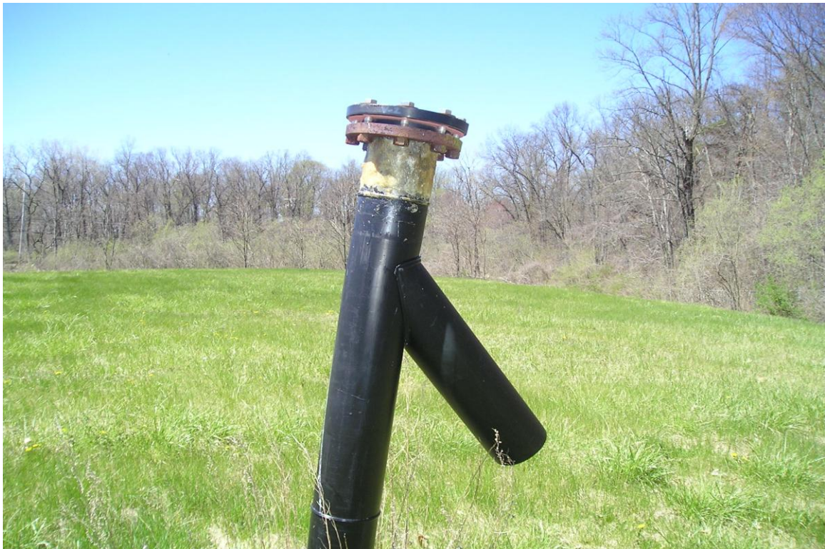
Photo 2: Vent V-2 (repair patch shown)
