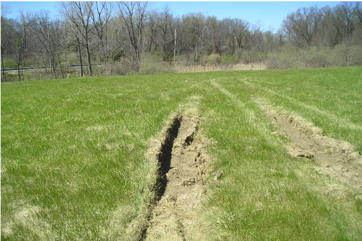
Photo 14: Ruts caused by vehicles carrying equipment
