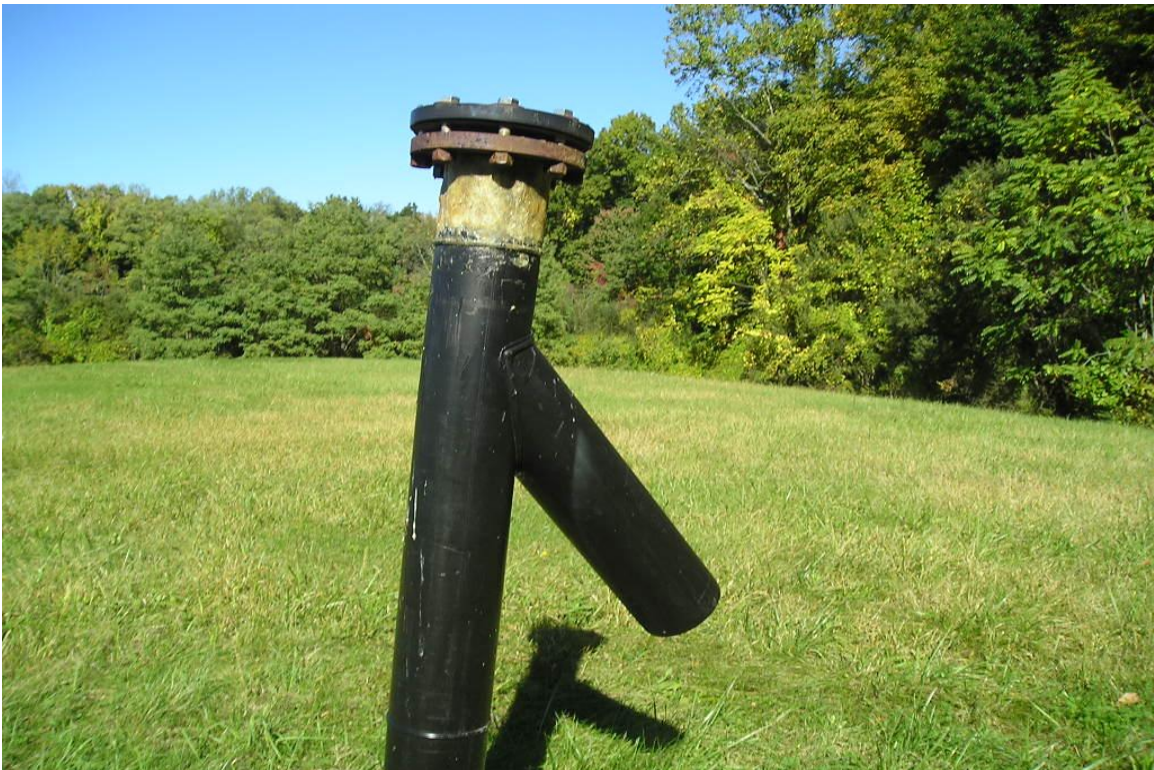
Photo 2: Vent V-2 (repair patch shown)
