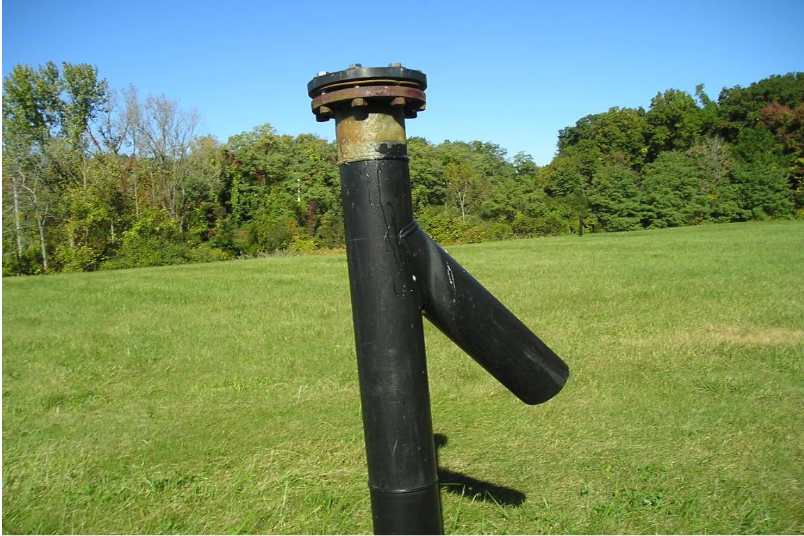
Photo 1: Vent V-1 (hole repair shown)
