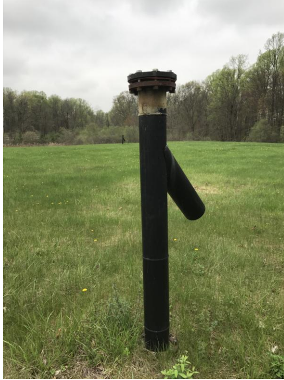
Photo 1: Vent V-1 (hole repair shown)
