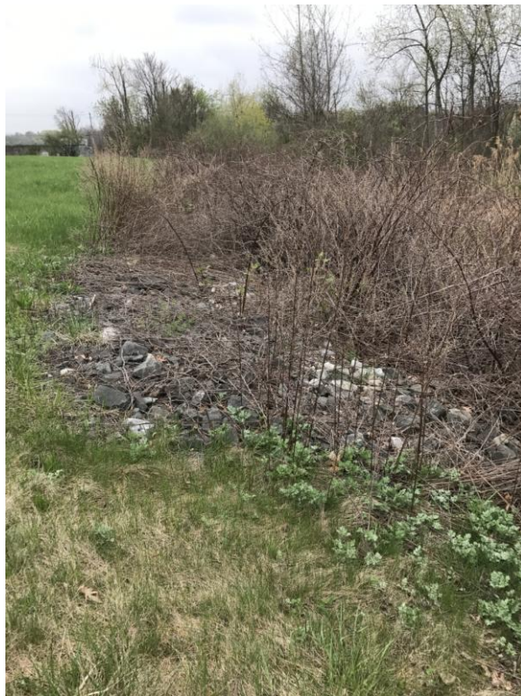
Photo 14: West slope area repair (looking south)
