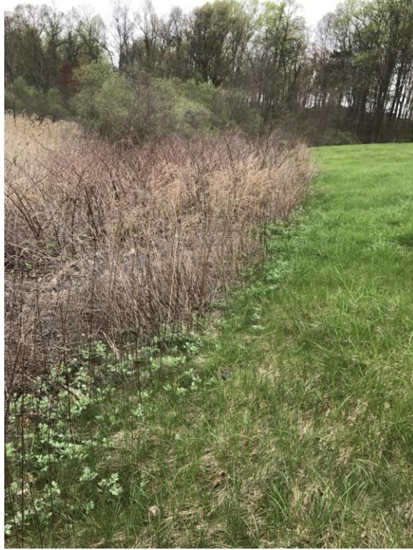
Photo 13: A portion of the west slope erosion area repair that needs to be cleared (looking north)
