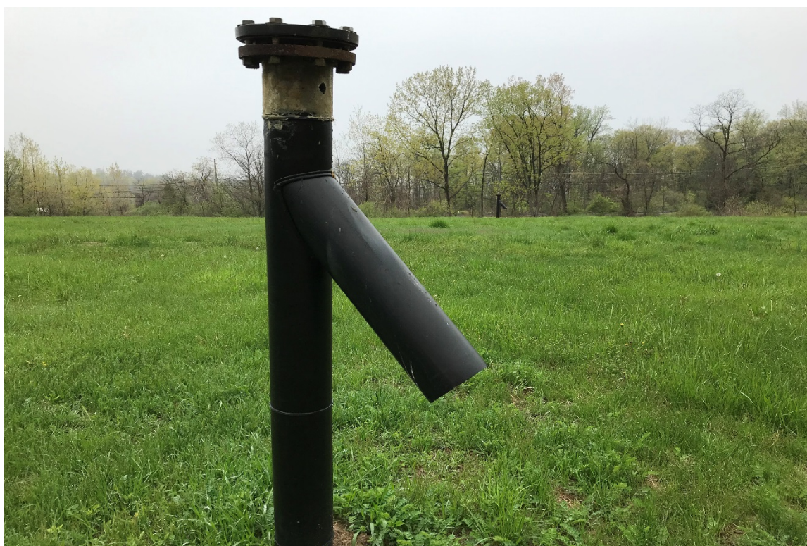
Photo 2: Vent V-2 (hole in repair patch shown)
