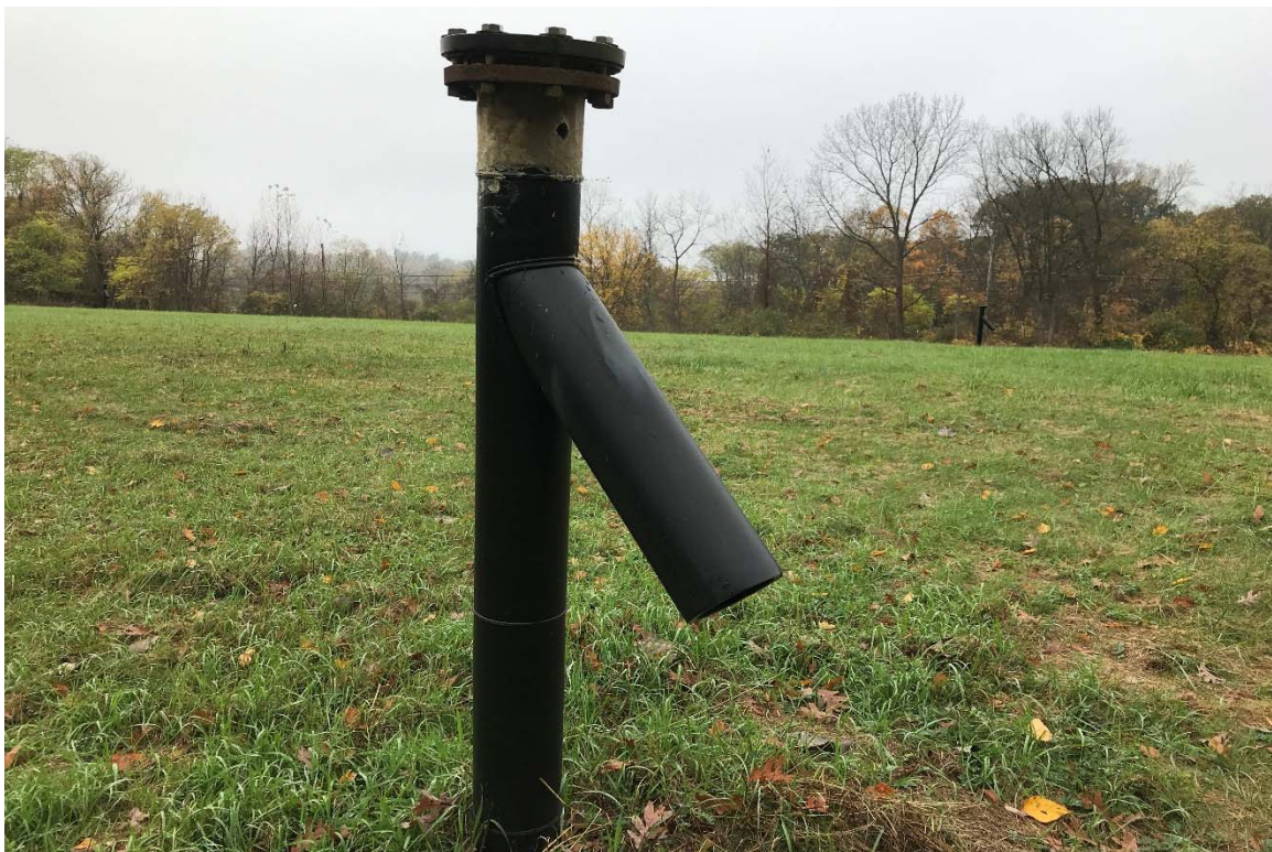
Photo 2: Vent V-2 (hole in repair patch shown)
