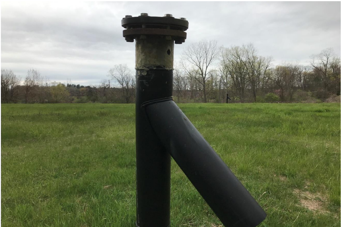
Photo 2: Vent V-2 (hole in repair patch shown)
