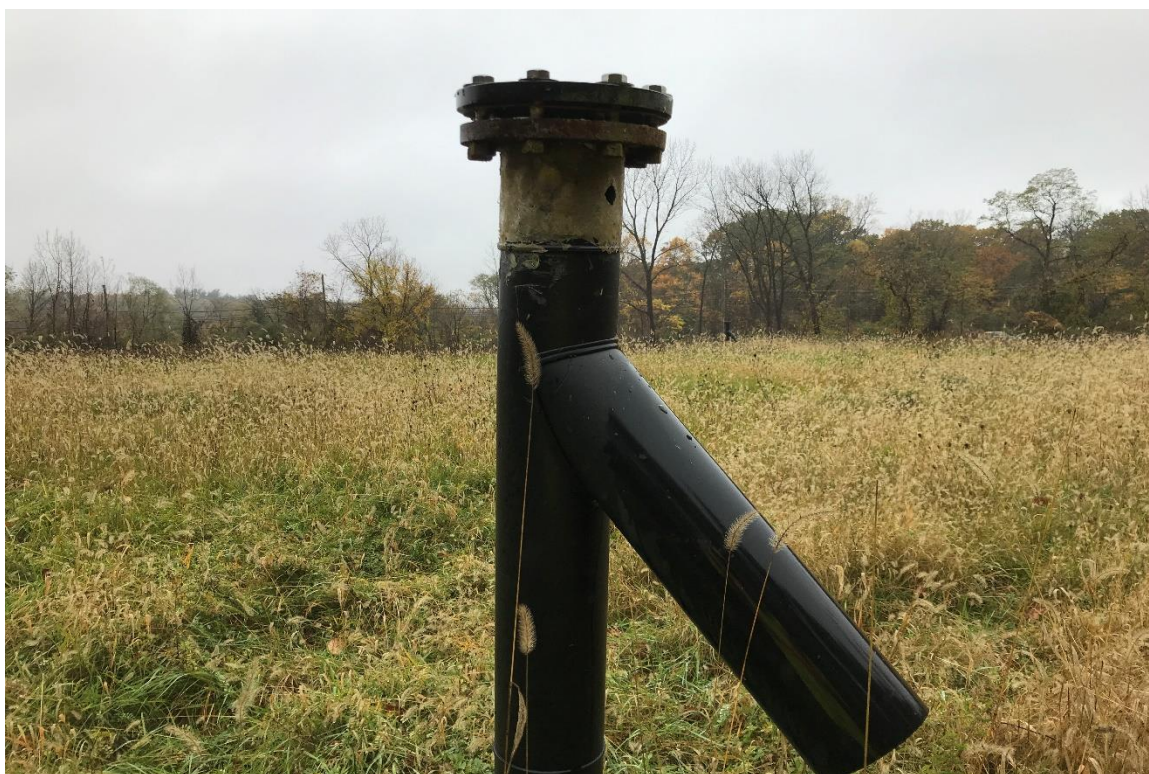
Photo 2: Vent V-2 (hole in repair patch shown)
