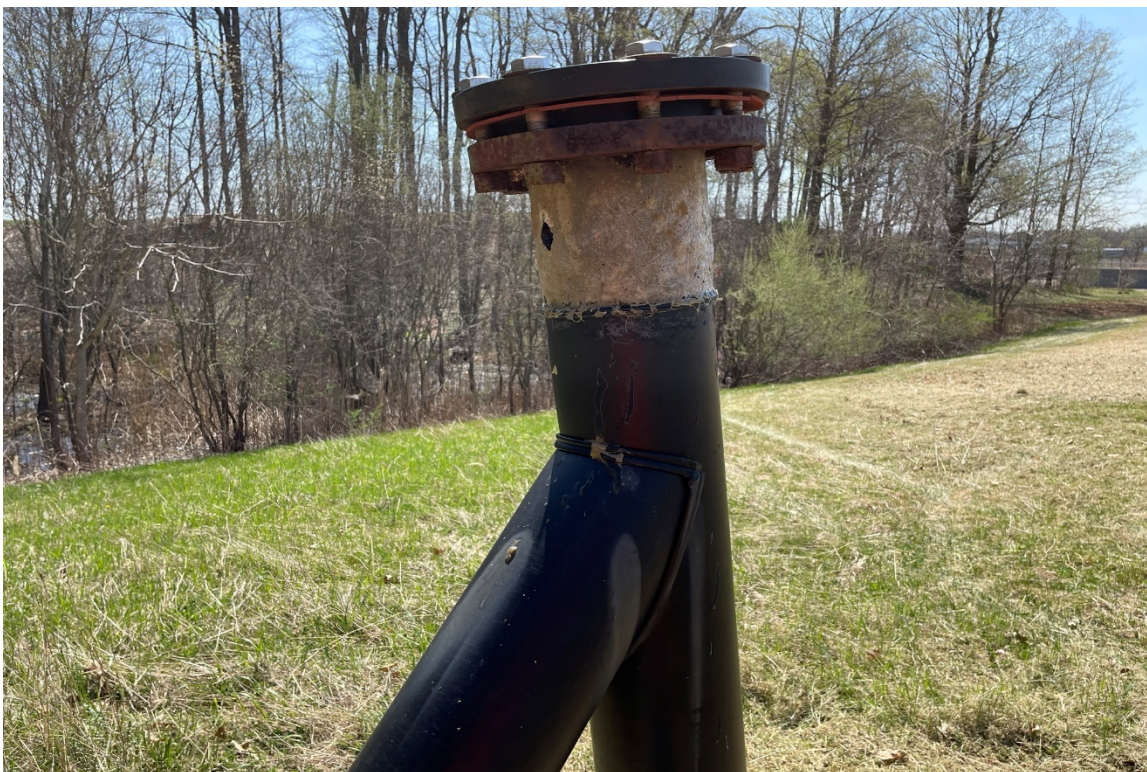
Photo 2: Vent V-2 (hole in repair patch shown)
