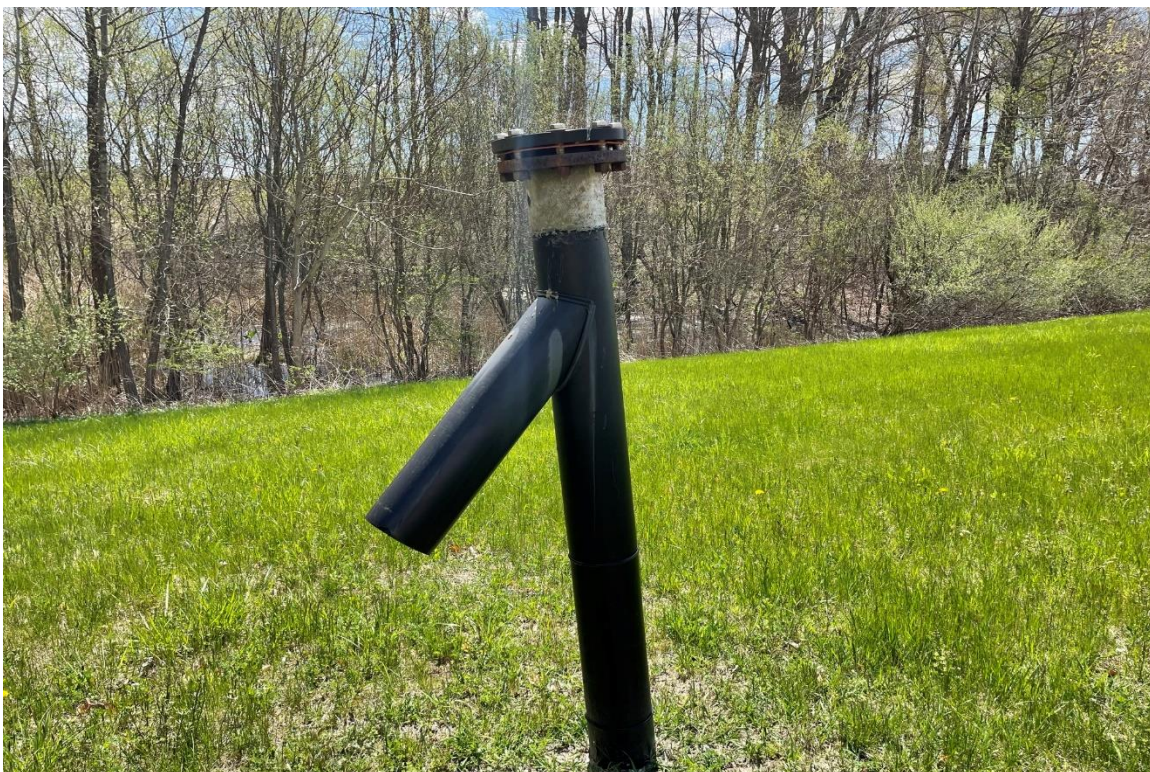
Photo 2: Vent V-2 (hole in repair patch shown)
