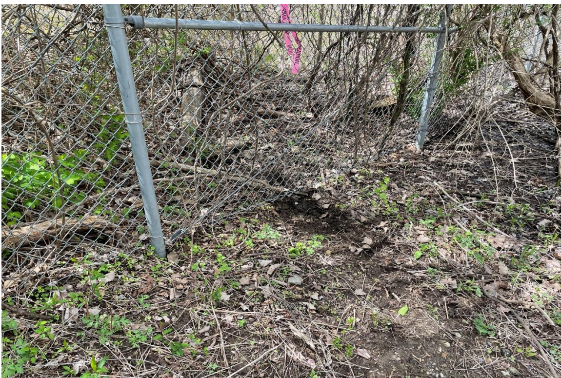
Photo 14: Animal burrow under south fence on landfill cap (looking southwest).
