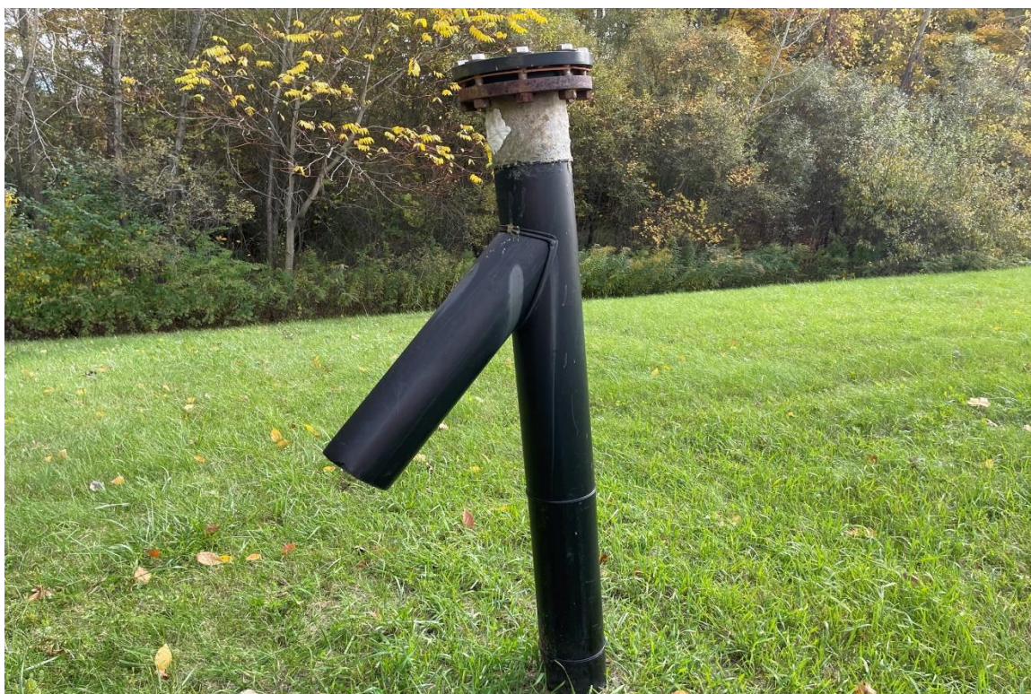
Photo 2: Vent V-2 (new repair patch shown)
