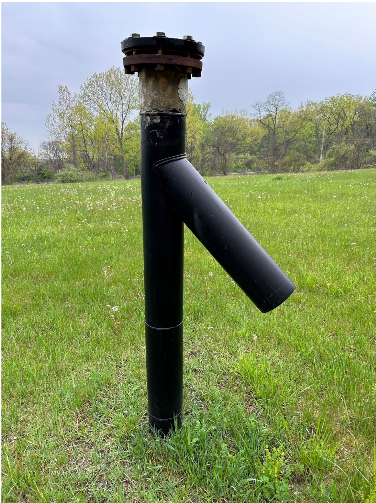
Photo 2: Vent V-2 (new repair patch shown)
