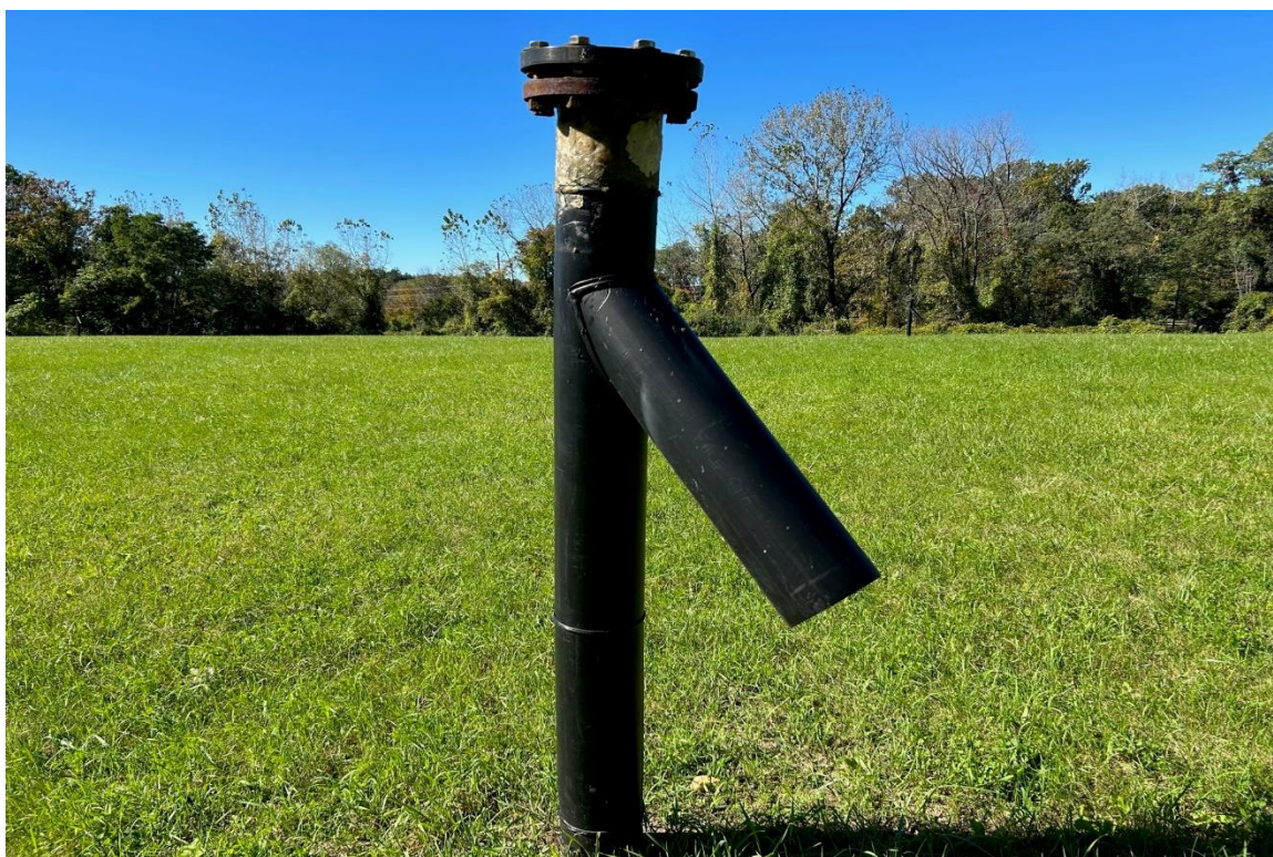
Photo 2: Vent V-2 (new repair patch shown)
