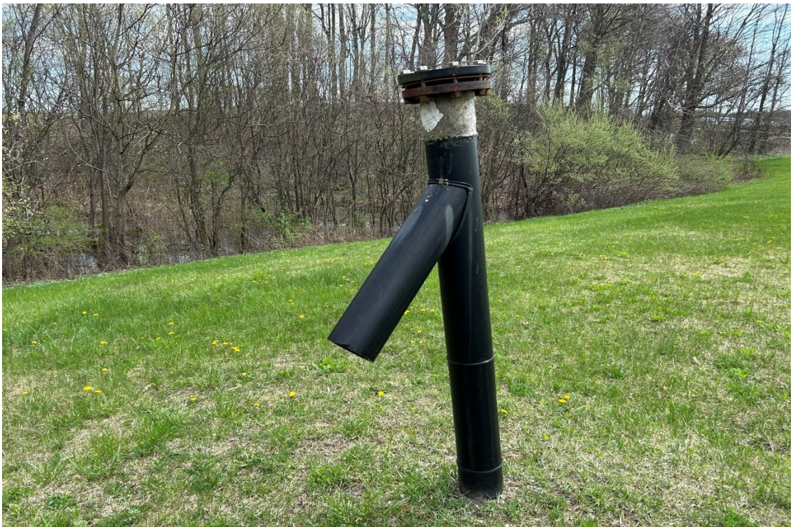
Photo 2: Vent V-2 (new repair patch shown)
