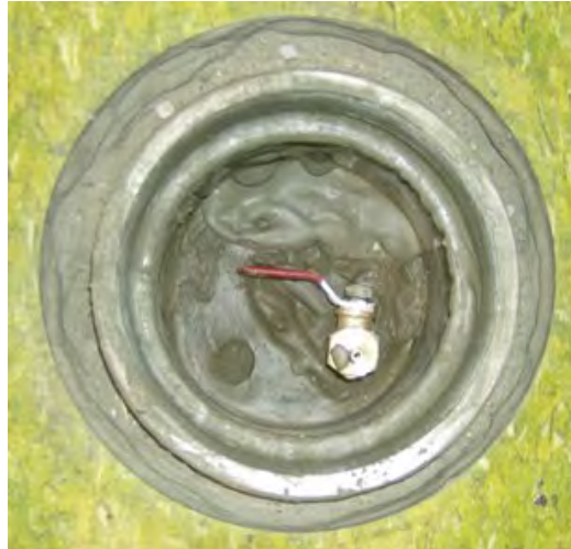
Photograph 1 - Overhead view of completed point via Flush-mount Well Cover Method
