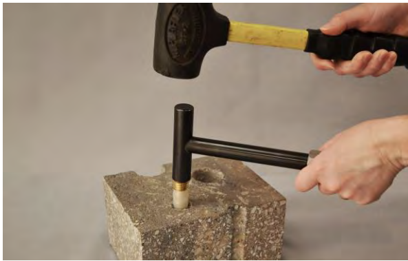
Figure 2. Installing the VAPOR PIN®
