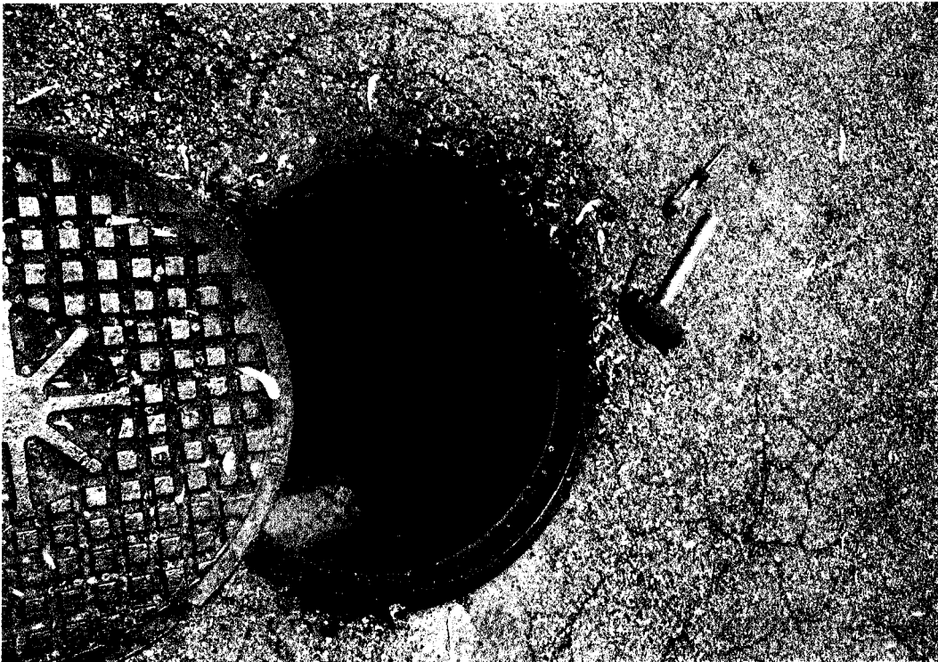
Figure 11 - Evaluation of the on-site catch basins and drainage systems.
