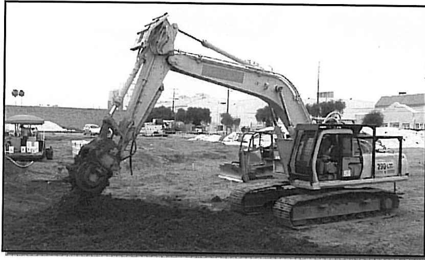
In-Situ Mixing of RegenOx™ On-Site
