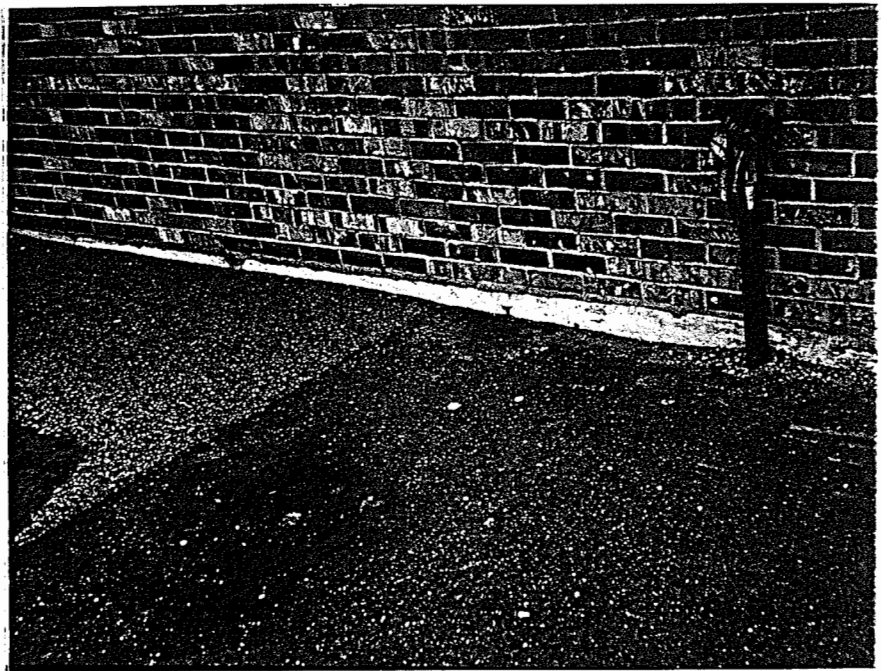
PHOTO 4. Fill port and vent pipe for UST located behind Van Tassel Cleaners.
