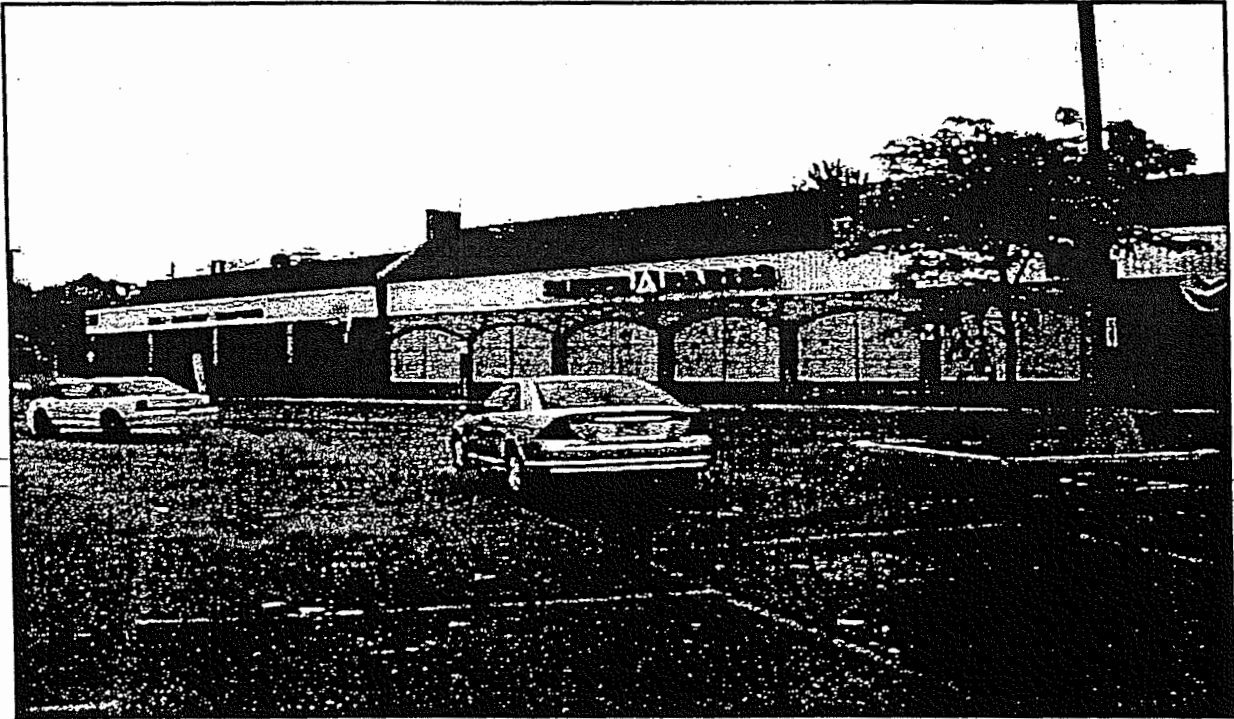
Photo 1 - Vacant supermarket building.
