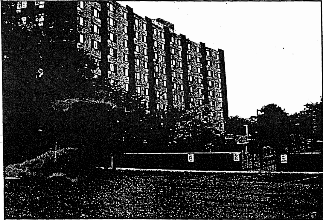
Photo 3 – Surrounding property – South of site.
