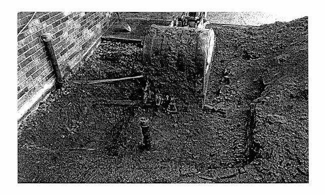
Overlying Soils Excavated to Expose Top of Tank
