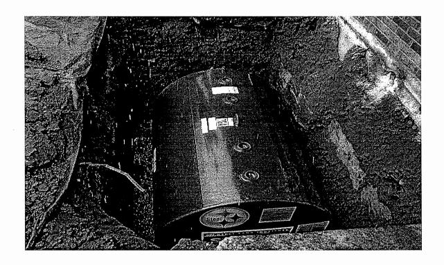
New Tank Installed in Excavation
