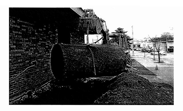
Removing Tank from Excavation
