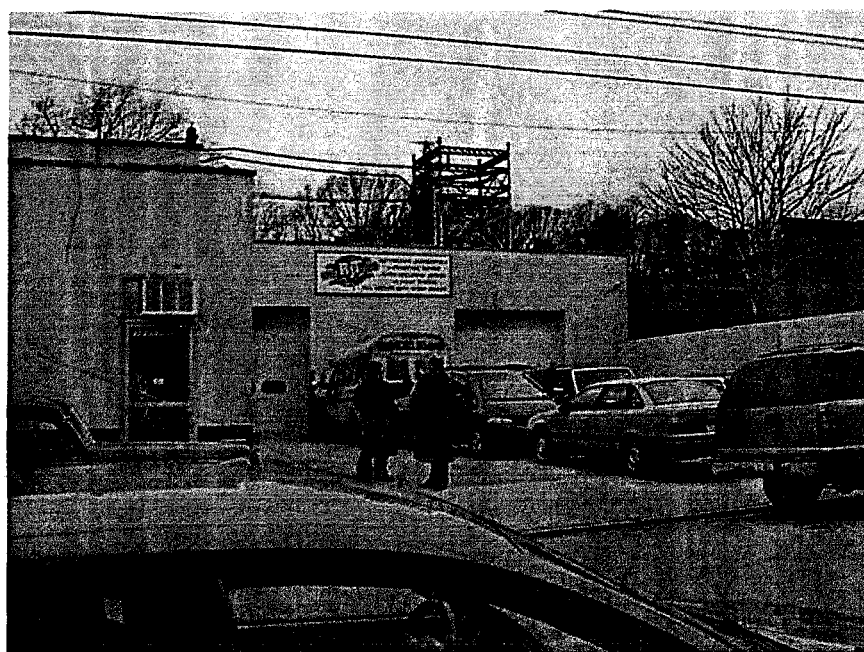
2. WEST VIEW OF THE ON-SITE BUILDING.
