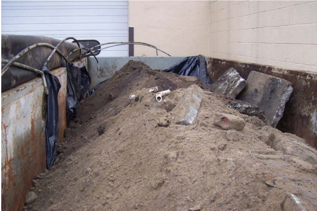
11. CONTAMINATED SOIL PLACED IN 20-CUBIC YARD ROLL-OFF CONTAINERS.
