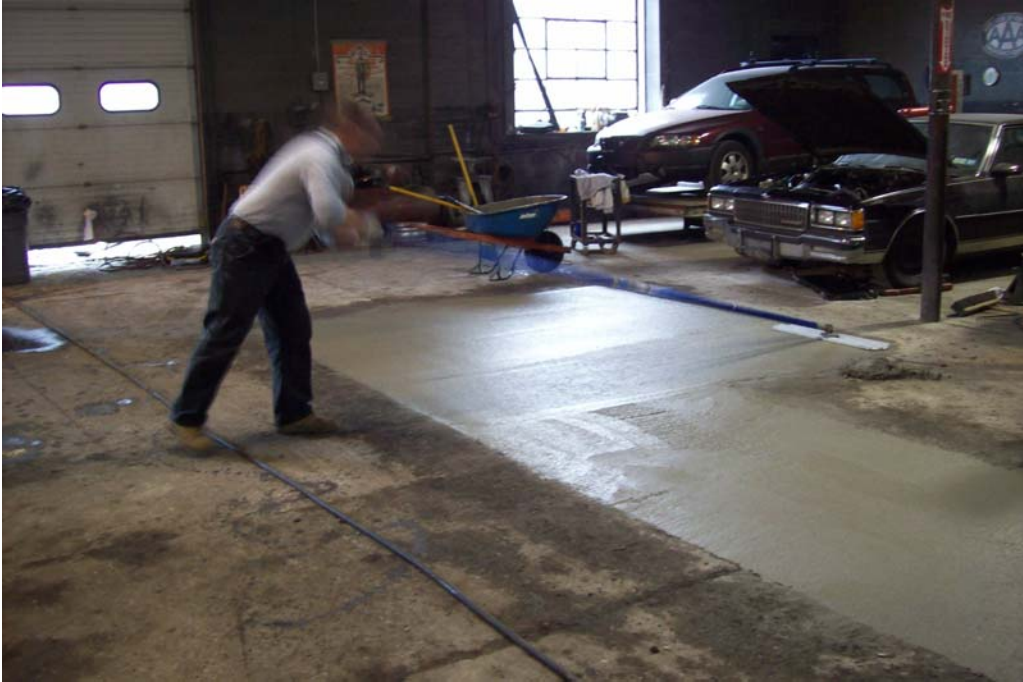
15. FINAL CONCRETE FLOOR RESTORATION.
