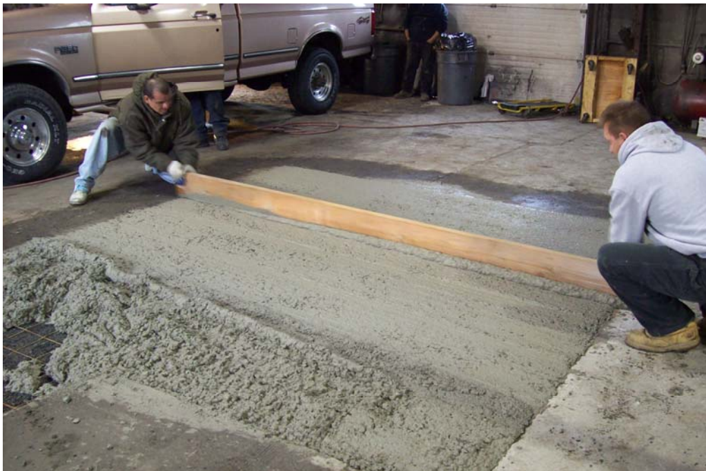
14. LEVELLING OF CONCRETE.
