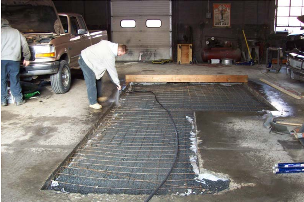
12. INSTALLATION OF 6X6 INCHES WIRE MESH PRIOR TO CONCRETE POURING.
