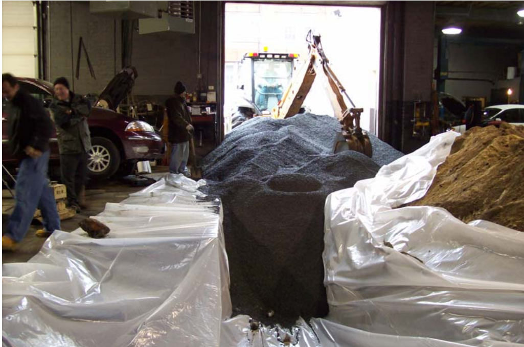
6. BACKFILLING WITH COARSE AGGREGATE TYPE 1 A CRUSHED STONES.
