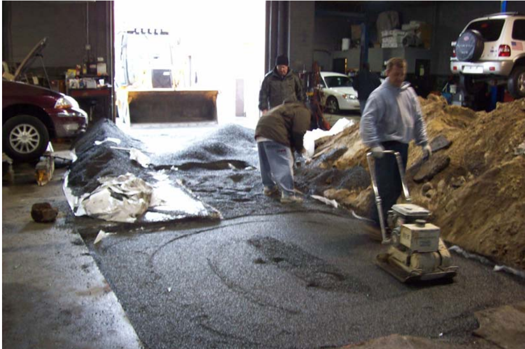
9. FINAL COMPACTION OF BACKFILL MATERIAL.
