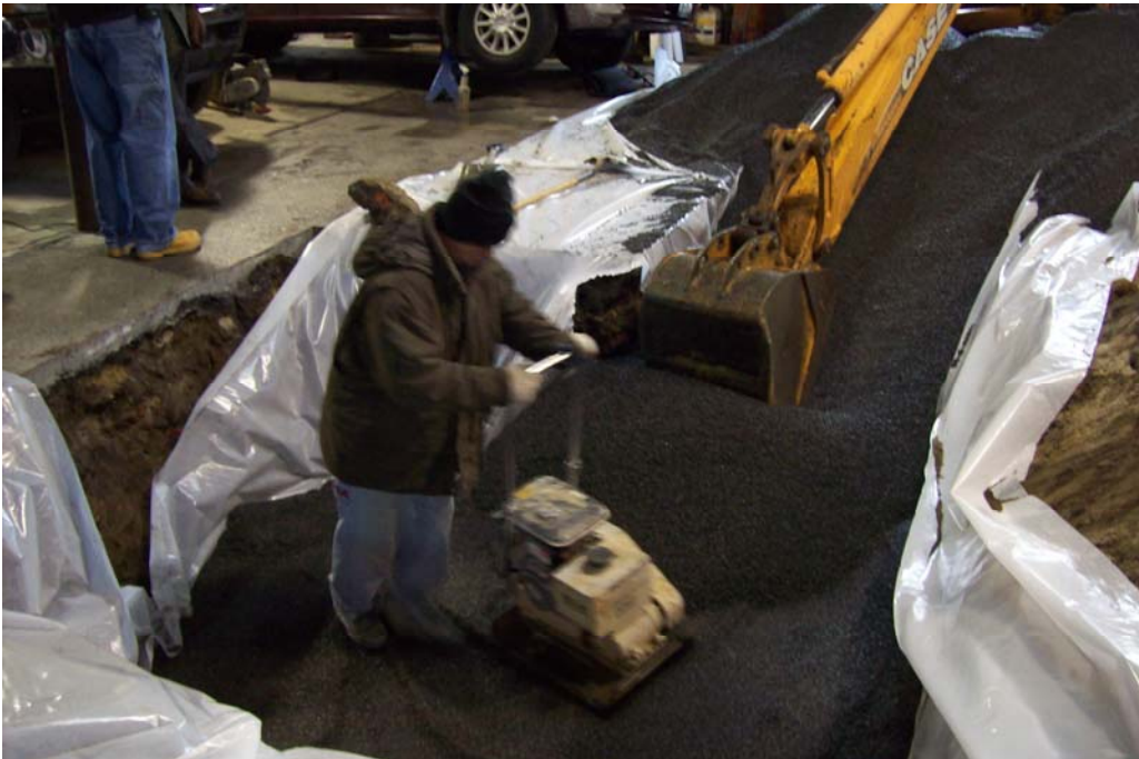
8. CONTINUOUS COMPACTION OF BACKFILL MATERIAL.
