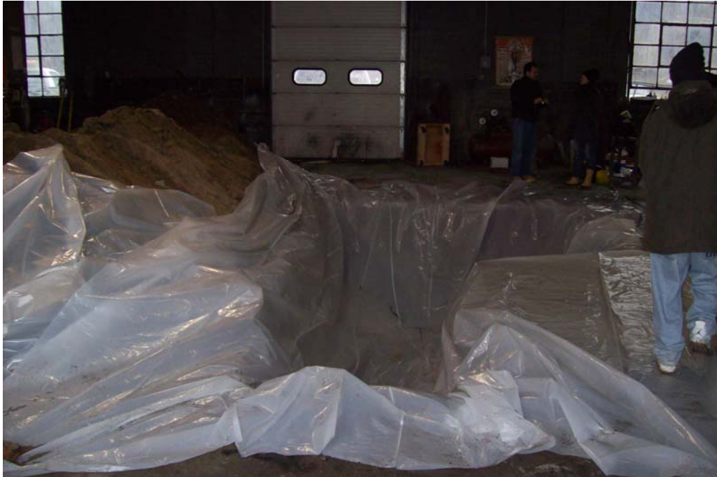
5. 1 LAYER OF 6-MIL POLYERHYLENE SHEETING ON TOP OF EXCAVATED SOIL PRIOR TO BACKFILLING.
