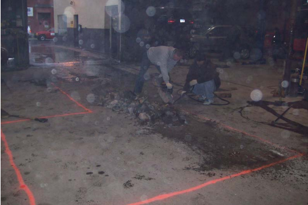
1. SAW CUT OF CONCRETE FLOOR.
