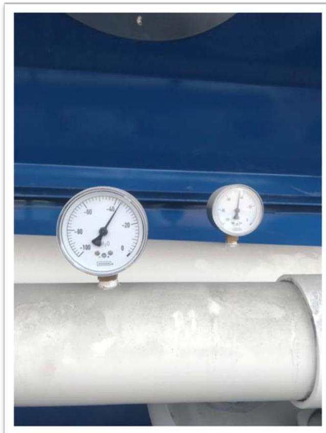
**8. Vacuum Gauges of the SVE System Unit after System Maintenance**
