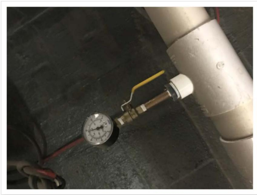
**6. Vacuum Gauge of the SVE System in the Repair Shop Area**
