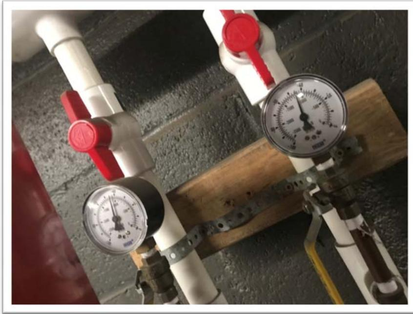
**5. Vacuum Gauges of the SVE System in the Repair Shop Area**
