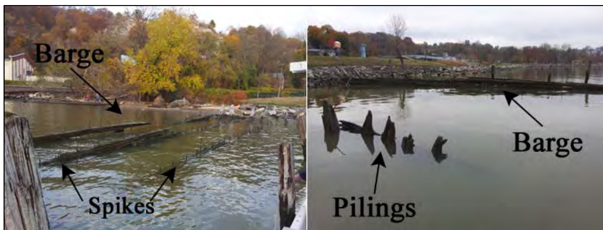
Figure 3. Left –Partially submerged barge. Note metal spikes at and just below the waterline. Right – Looking south from within the IMPACT site showing the partially submerged barge as well as exposed pilings near the debris field.
