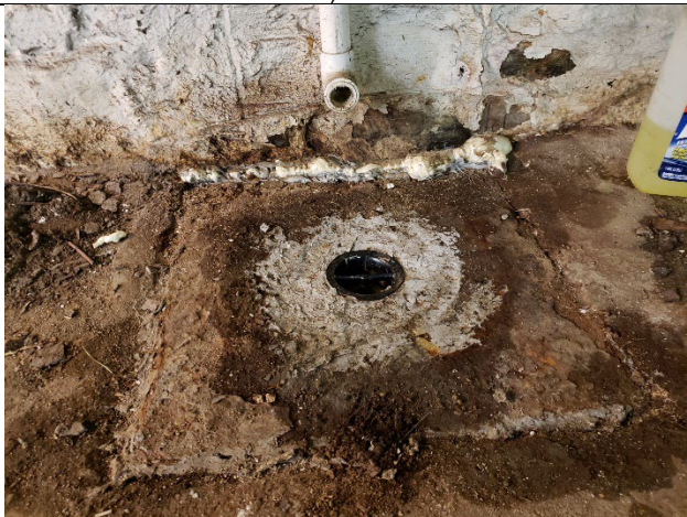
One-way drain valve (black circle at center) re-installed at brick sump in basement at 49 Main St.
