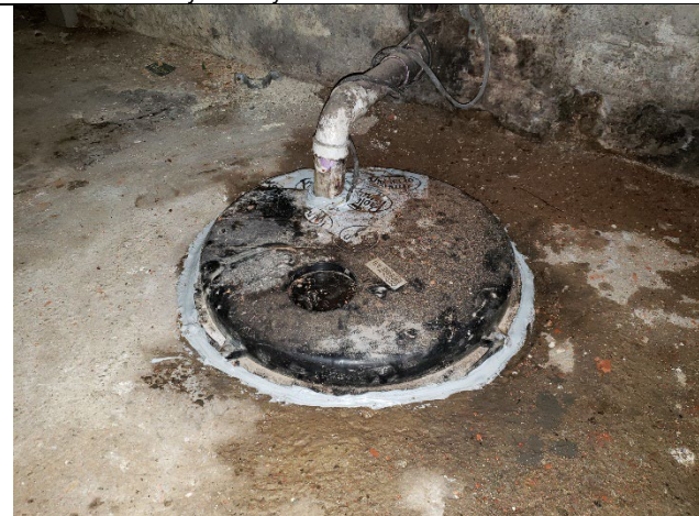
Re-sealed sump cover at DW-02
