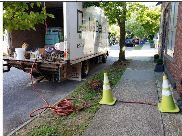
Injection equipment staged in LaBella box truck on N. Dutcher St.; hose entering basement through conduit access point at street level.
