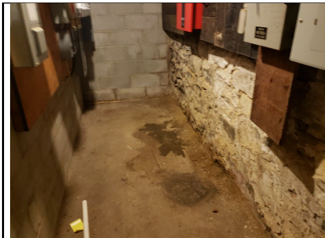
Leaking from slab (likely at connection with field stone wall) in utility hallway in basement at 49 Main St.
