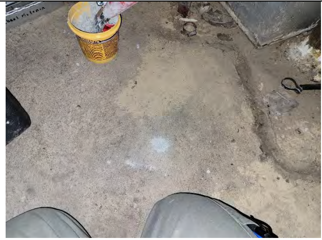
Photograph 34: Filled Temporary Vapor Pin Installation hole at Location SSV/IA-2
