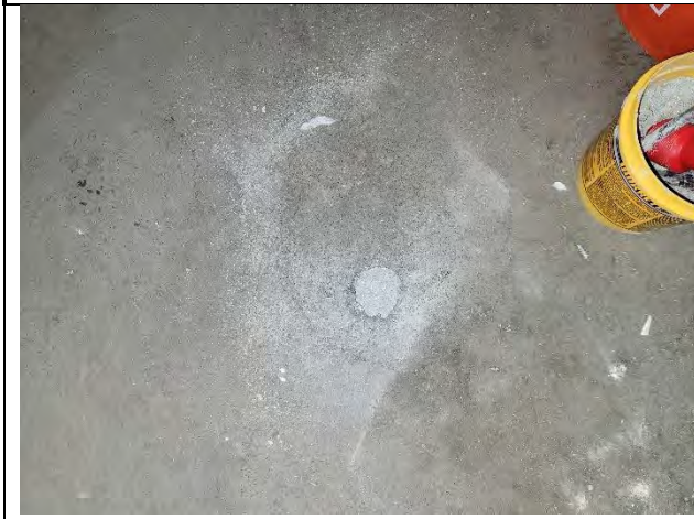
Photograph 33: Filled Temporary Vapor Pin Installation hole at Location SSV/IA-1
