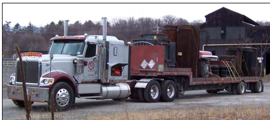
Photo 1: Removal of PCB Contaminated Transformers and Fluid
