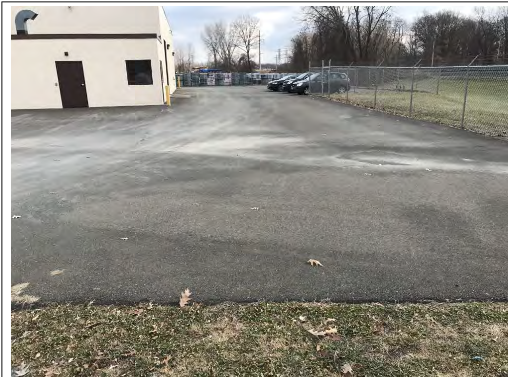
Photograph #7 – View from the western portion of MERECO property looking east. View shows a small crack extending from the southeastern corner of the MERECO building. The crack had been filled with sealant/crack-filler
