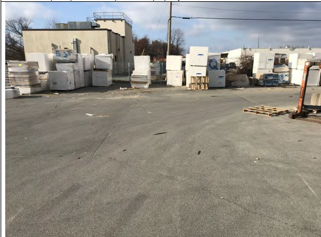
Photograph #20 – View from the western portion of Allied property looking west. View shows the asphalt pavement cap on Allied property.
