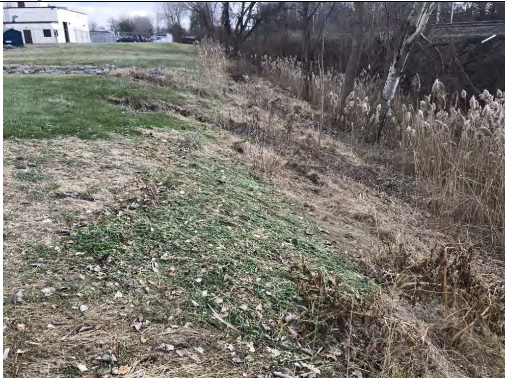
Photograph #16 – View from the southeastern portion of the MEREKO-owned property looking east. View shows two eroded areas on the slope.
