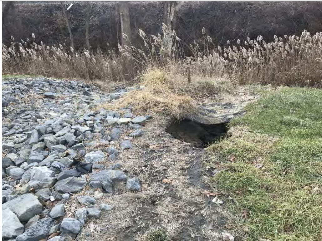
Photograph #18 – View from the southern portion of the MEREKO-owned property looking south. View shows a previous repair (riprap area) on the left-hand side of the photograph and the eastern erosion area on the right-hand side of the photograph, respectively.
