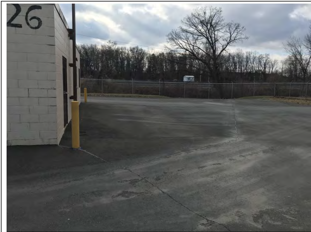
Photograph #5 – View near the northwestern corner of the MERECO building looking south. View shows a small crack extending from the northwest corner of the MERECO building, and a slight separation of a pavement joint extending towards the letdown channel in the background of the photograph. Both had been filled with sealant/crack-filler.
