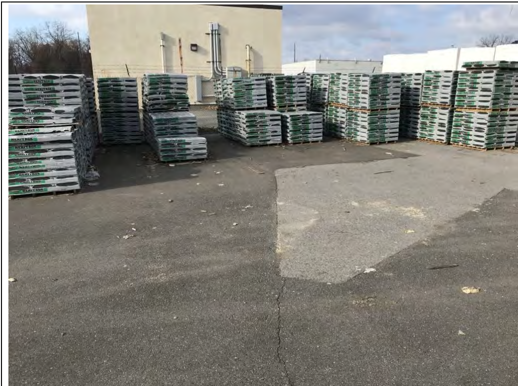
Photograph #23 – View from the western portion of Allied property looking east. View shows a small crack and a slight separation at the edge of the asphalt pavement cap on Allied property.
