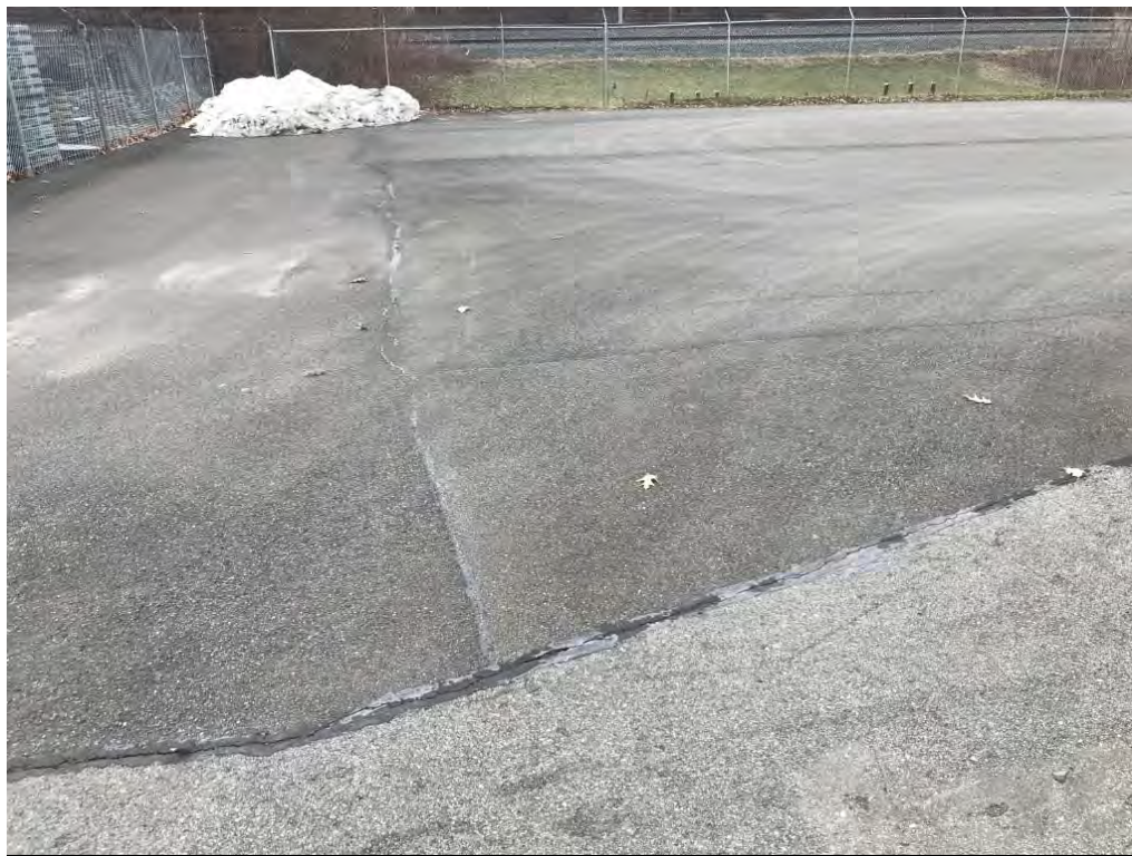
Photograph #2 – View from the eastern edge of MERECO property looking south. View shows a slight separation of a pavement joint filled with sealant/crack-filler
