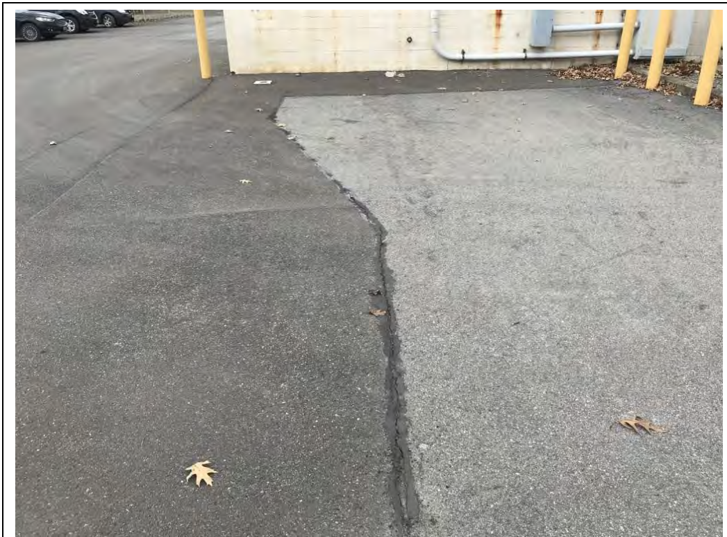
Photograph #1 – View from the eastern edge of MERECO property looking west. View shows a slight separation of a pavement joint filled with sealant/crack-filler.
