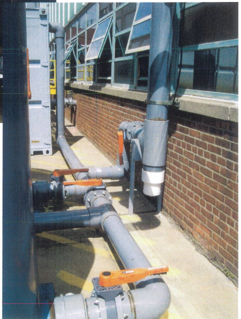
Photographs 9 and 10. Building 20/25 Type B SSDS discharge piping.
