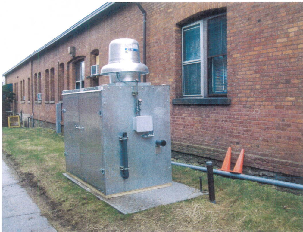
Photograph 3. Initial placement of Type A SSDS at Building 21.
