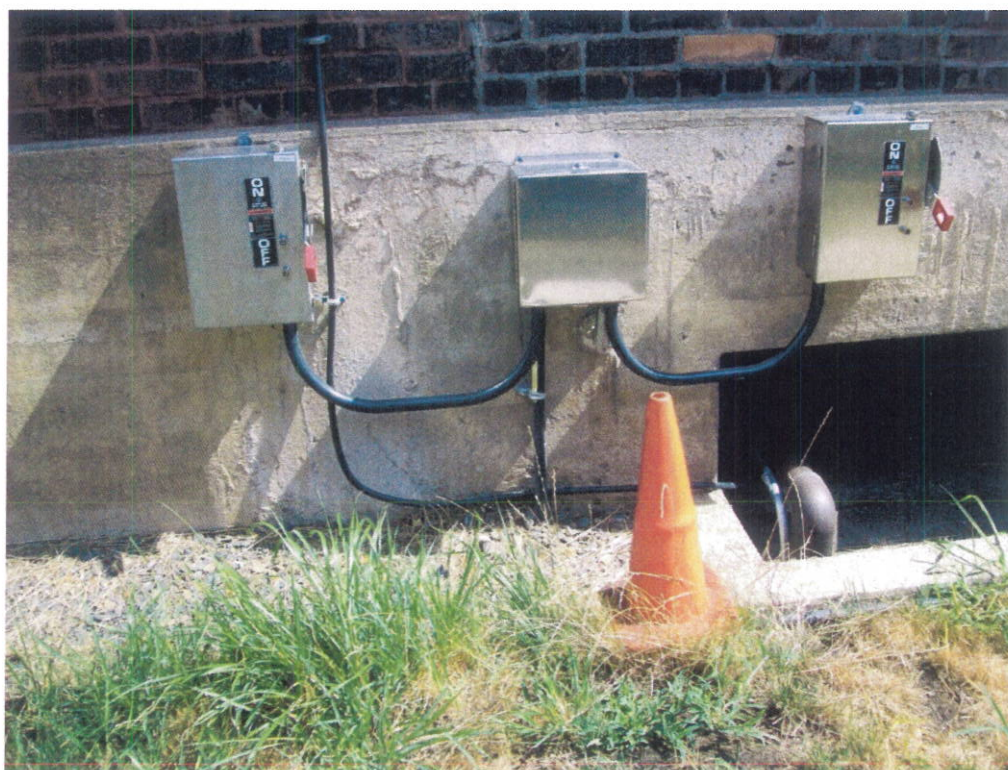
Photograph 3. Initial placement of Type A SSDS at Building 21.
