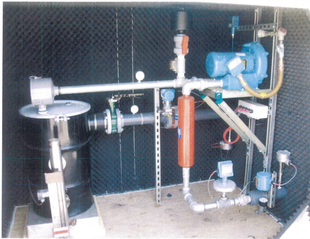
Photograph 3. Type A SSDS enclosure contents (Building 114).
