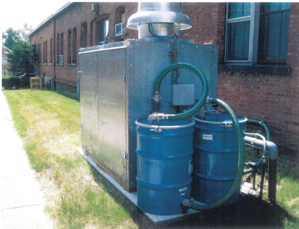
Photograph 5. Completed Building 21 Type A SSDS.
