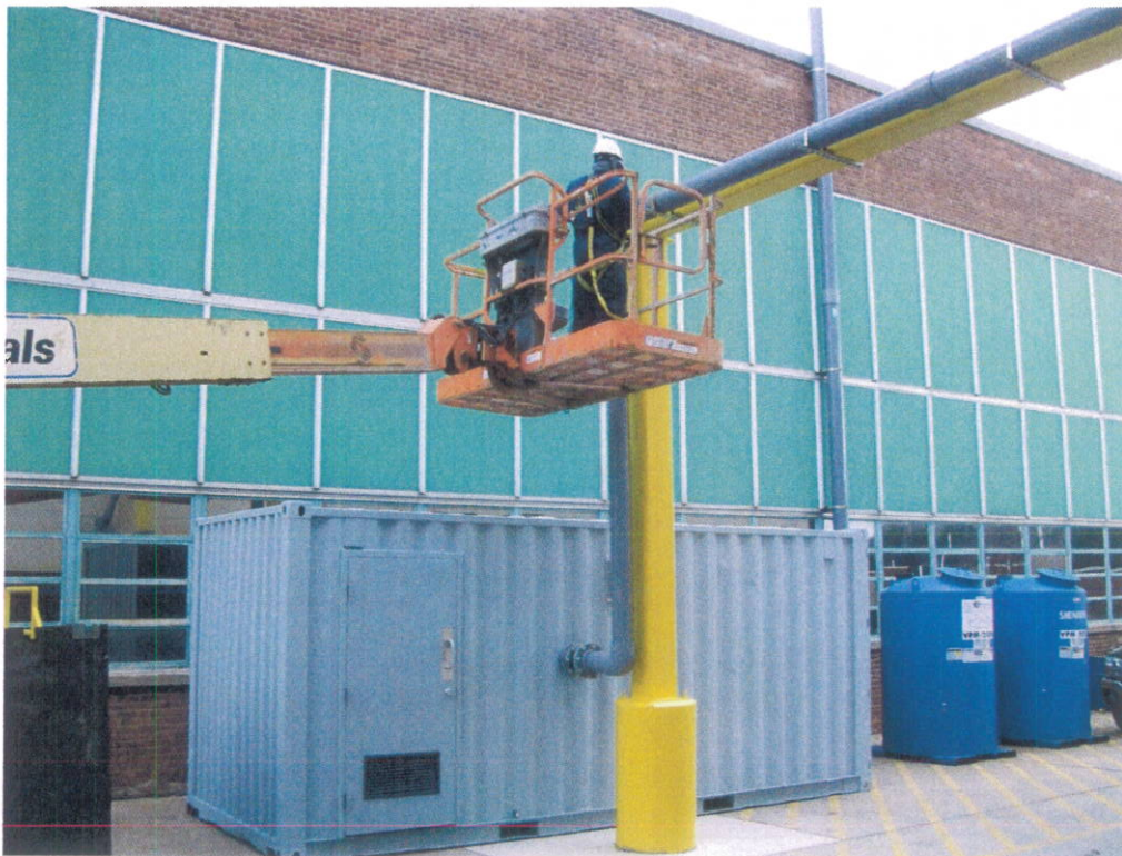
Photograph 8. Securing Building 25 suction line to pipe bridge. Type B SSDS and carbon vessels in background.
