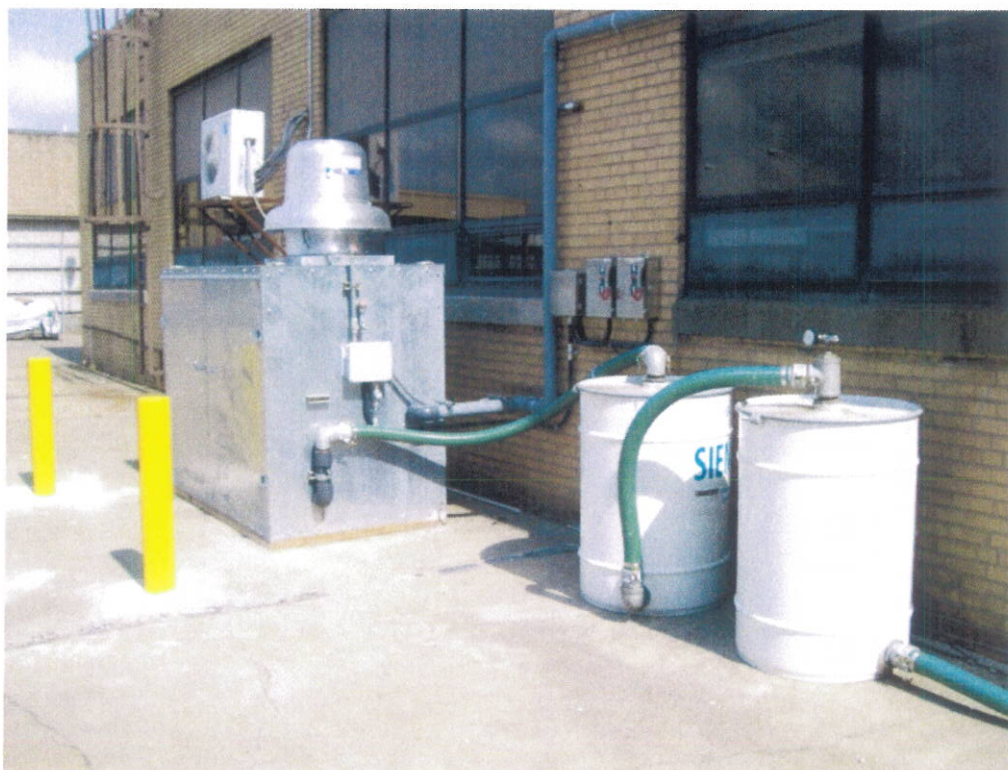
Photograph 6. Completed Building 114 Type A SSDS.
