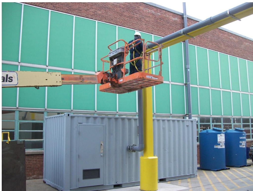
Photograph 8. Securing Building 25 suction line to pipe bridge. Type B SSDS and carbon vessels in background.
