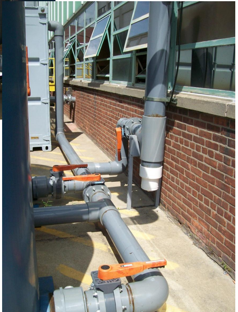
Photographs 9 and 10. Building 20/25 Type B SSDS discharge piping.
