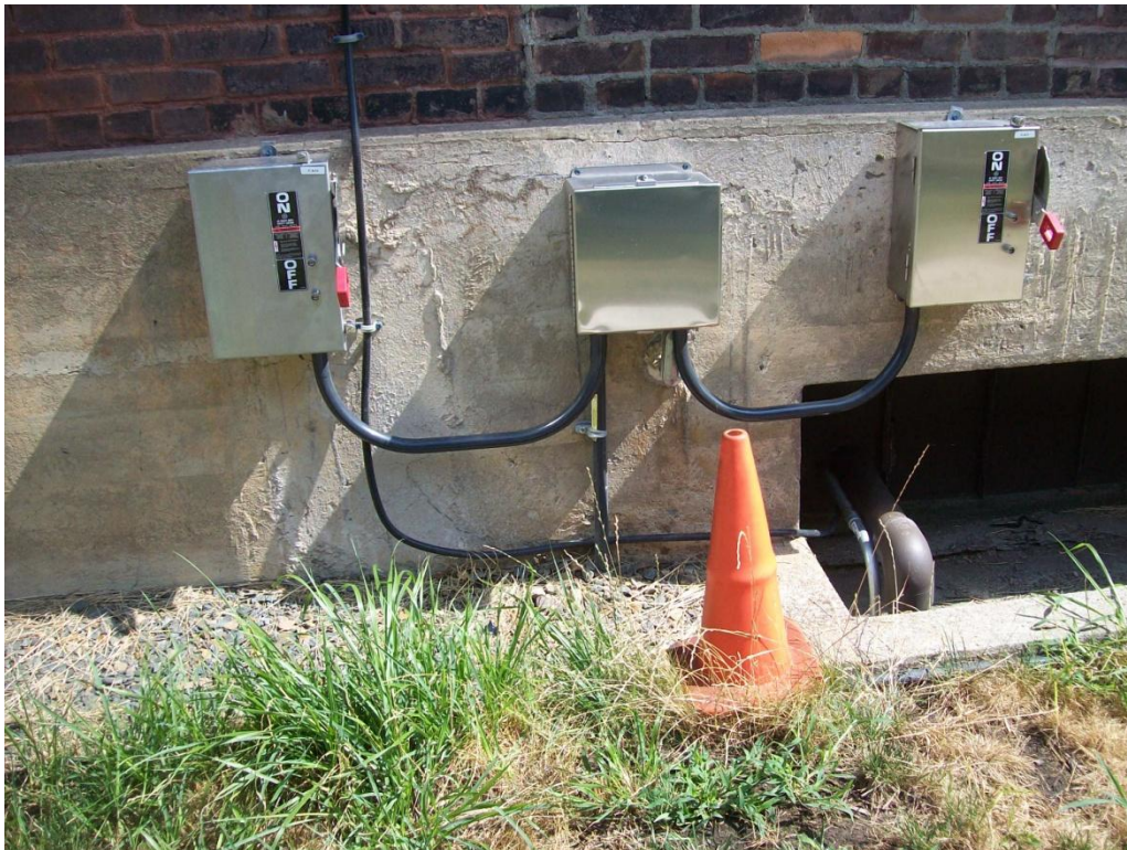
Photograph 3. Initial placement of Type A SSDS at Building 21.
