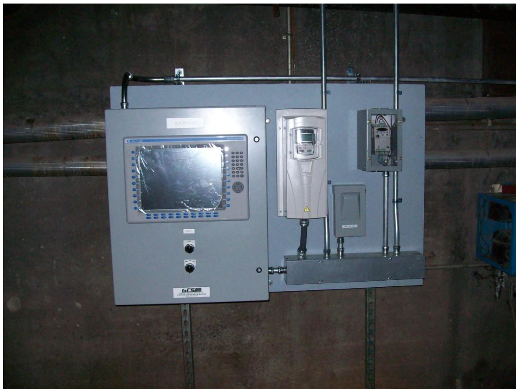
Photograph 4. Remote-mount control panel for Type A SSDS (Building 21 installation shown).
