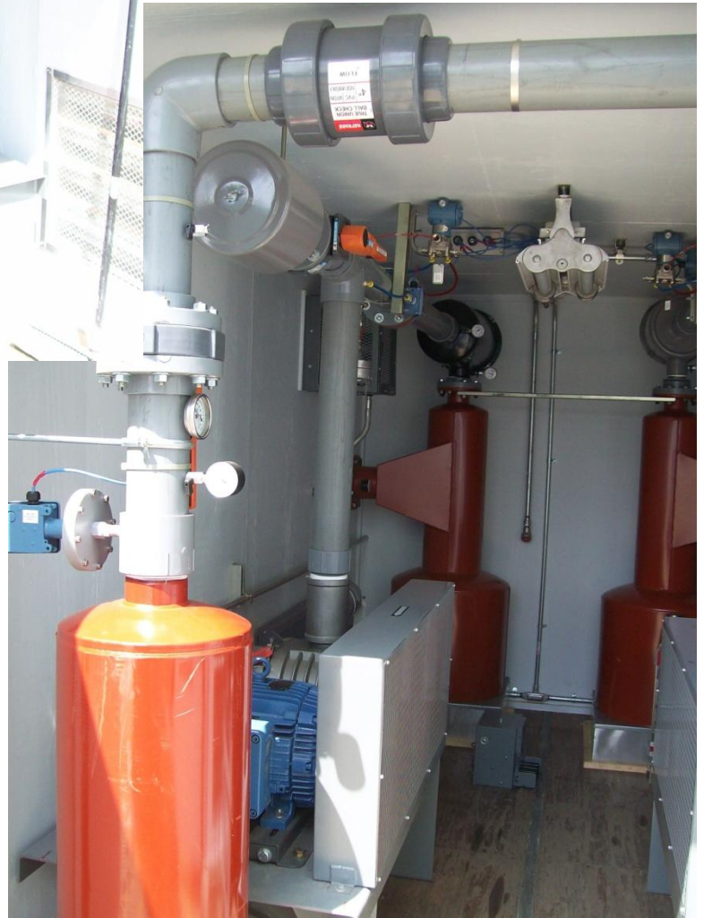
Photographs 11 and 12. Building 20/25 Type B SSDS mechanical room enclosure contents.
