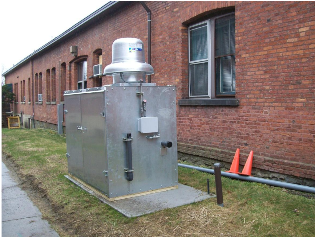
Photograph 3. Initial placement of Type A SSDS at Building 21.
