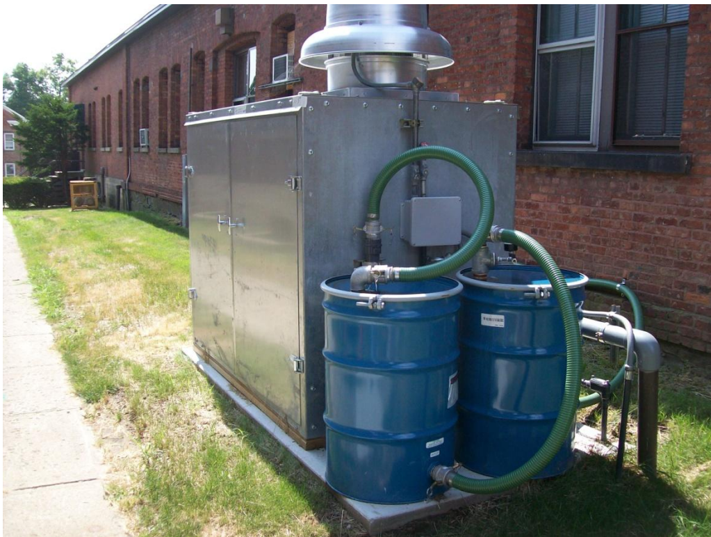
Photograph 5. Completed Building 21 Type A SSDS.
