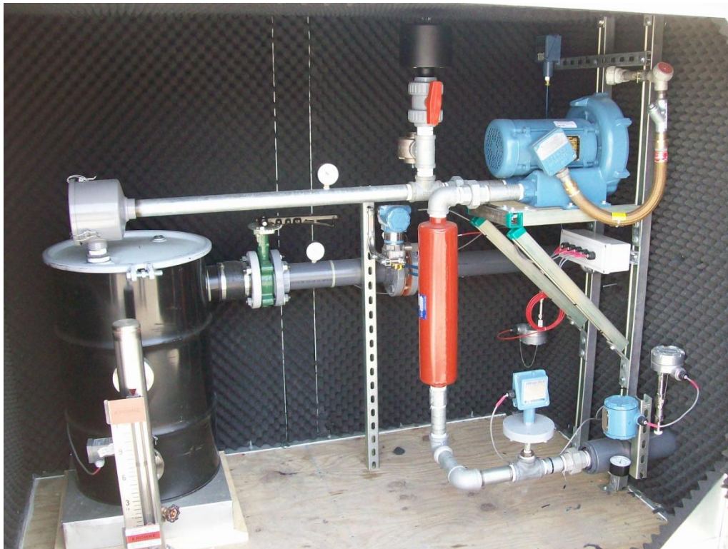
Photograph 3. Type A SSDS enclosure contents (Building 114).
