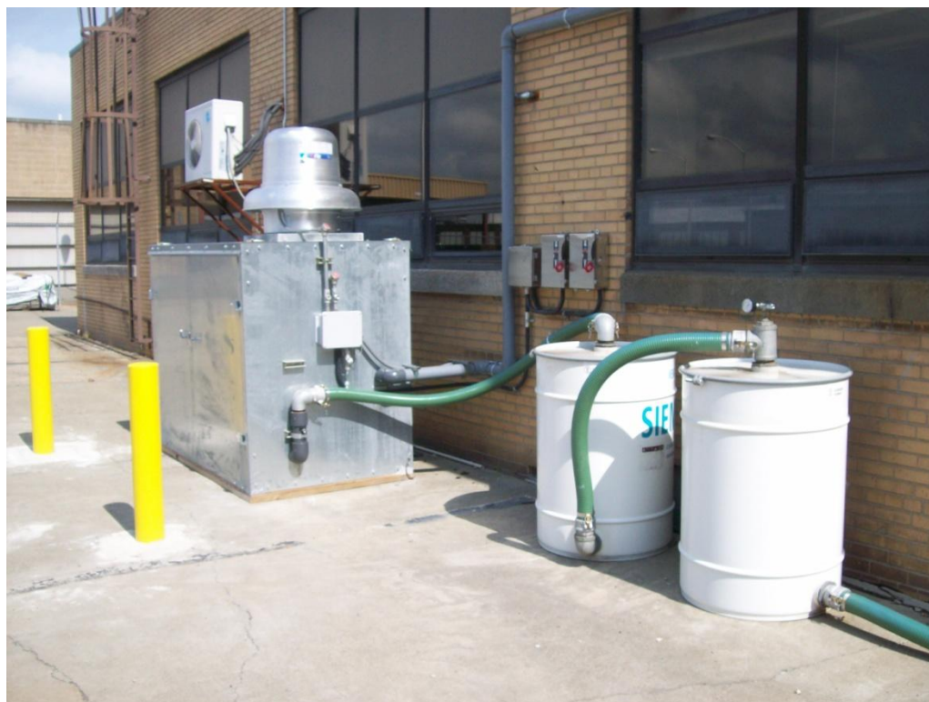
Photograph 6. Completed Building 114 Type A SSDS.
