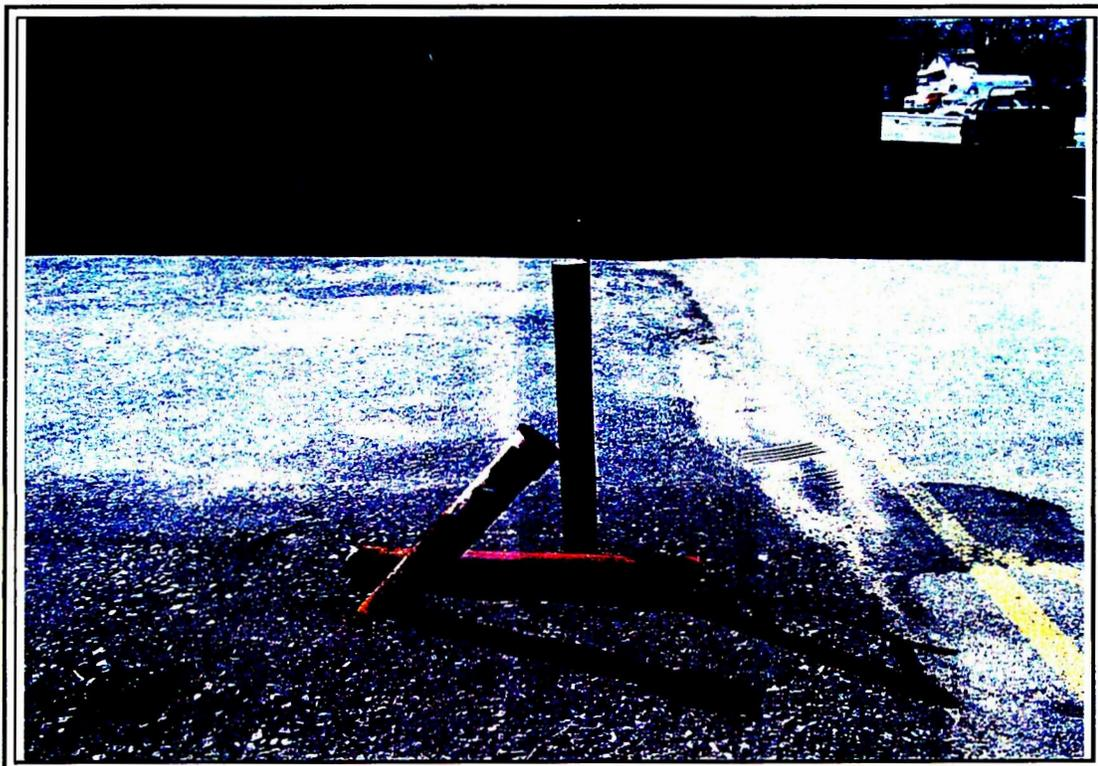
**Photograph 2.** Damaged protective bollard for MW-1 located at northwestern corner of the paved parking area between Buildings 14 and 16.
