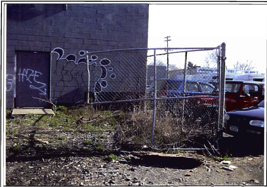
Photograph 1. Damaged access gate on east end of site with missing fencing on the lower left hand side of the gate.
