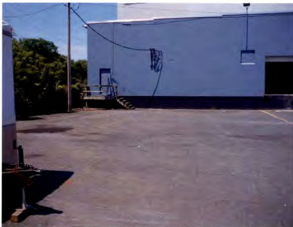
Photograph 11: Photo looking southwest showing paved area between Buildings #14 and #16 in good condition.
