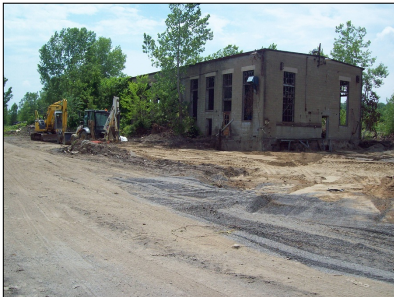
Photograph 4: Placement of clean fill at remediated North Power Station, OU-1 (July 2009).
