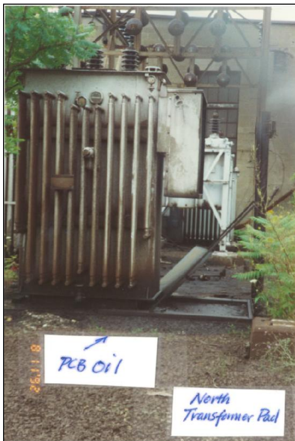
Photograph 1: Leaking transformer at the North Power Station prior to removal (August 1992).
