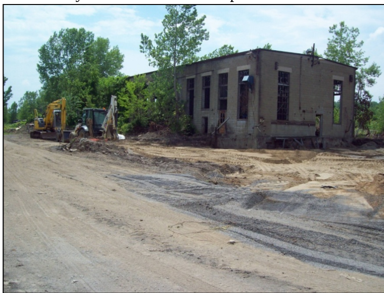
Photograph 4: Placement of clean fill at remediated North Power Station, OU-1 (July 2009).
