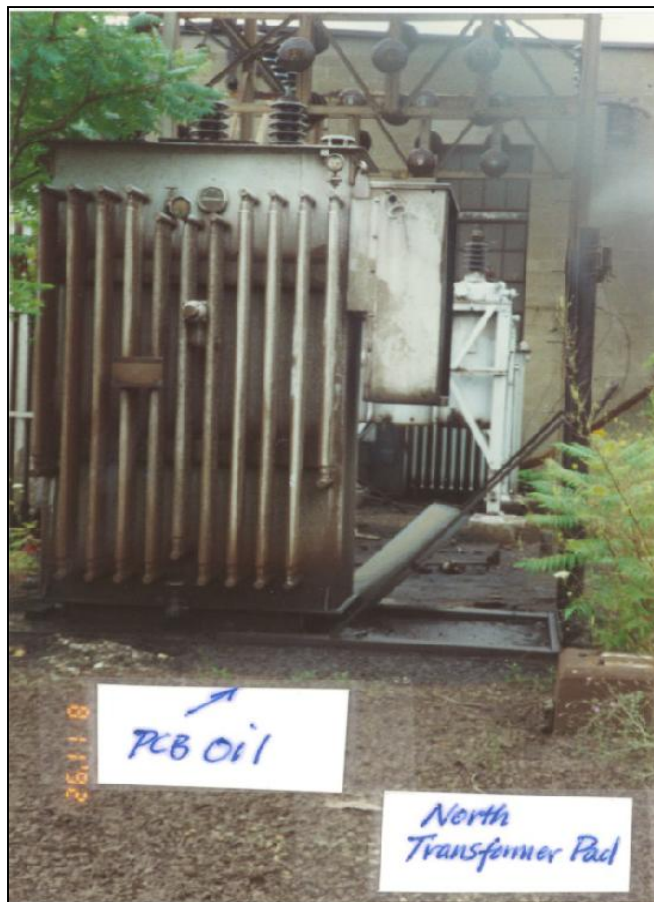
Photograph 1: Leaking transformer at the North Power Station prior to removal (August 1992).
