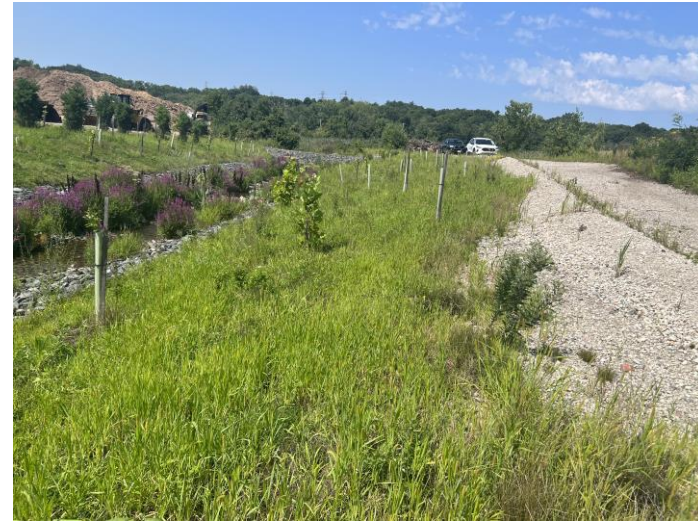
Photograph 4: View facing upstream of the riparian planting zone along the north side of the stream channel.
