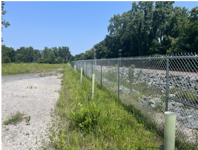
Photograph 23: Riparian planting zone along the newly installed chain-link fence.
