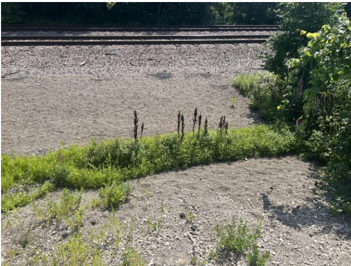
Photograph 15: Emergent wetland fill area 1.
