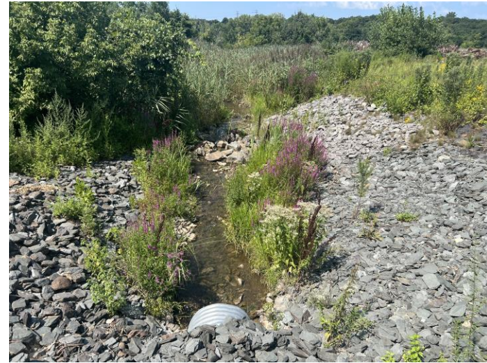
Photograph 6: View facing upstream at the upper portion of the site.
