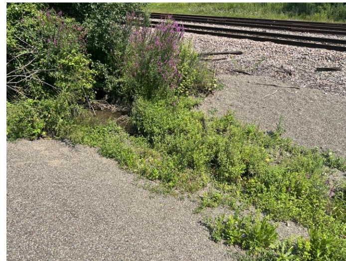
Photograph 26: Emergent wetland fill area 8.
