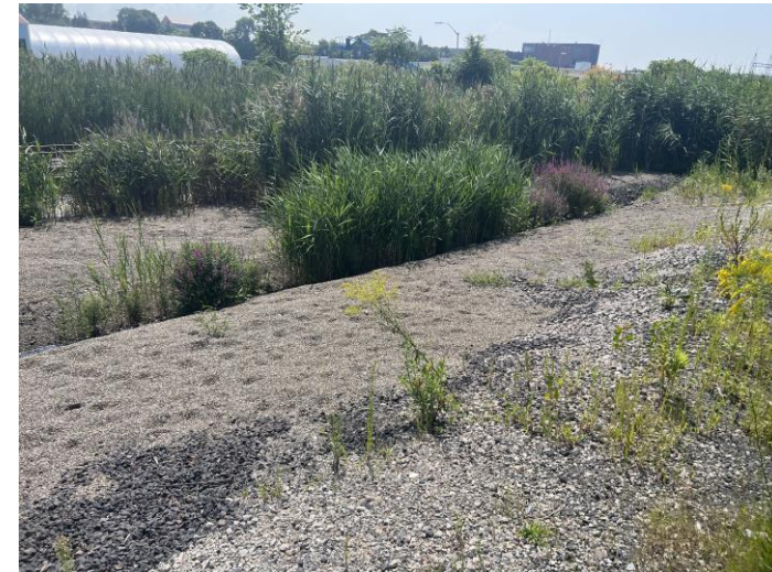
Photograph 20: Emergent wetland fill area 5.
