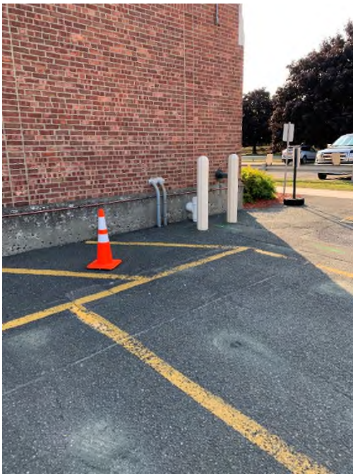
Picture 4: Lines coming out from building were untraceable. Direct connected and used dropped box method to locate lines.
