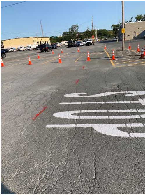
Picture 9: Electrical conduit running g along driveway
