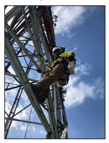
Personal fall arrest, fall restrain and fall limiting devices are critical when other fall protection systems do not exist.
